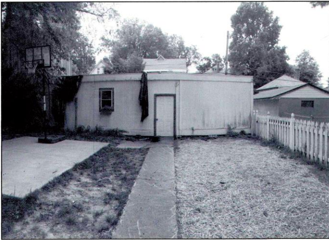
1408 HIGHLAND AVENUE: EXISTING GARAGE (TO BE REMOVED)
