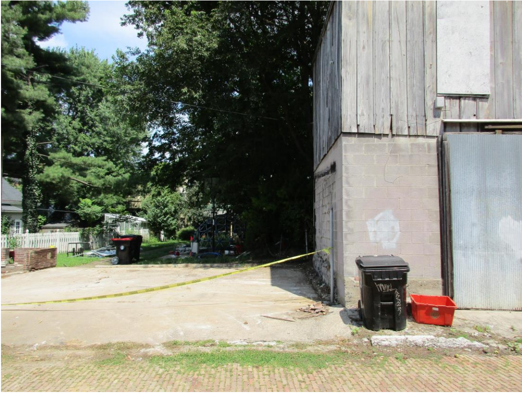
Looking north from alley/ Location of new garage
