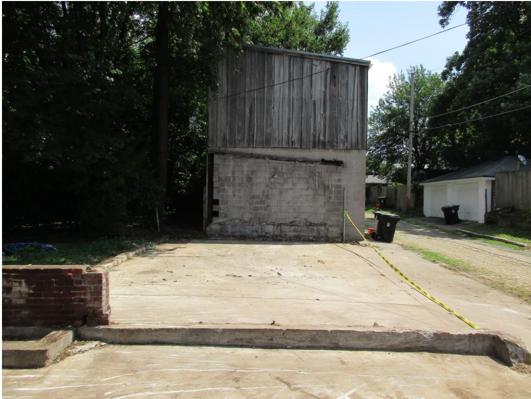
Looking east from west side of garage/ Location of new garage
