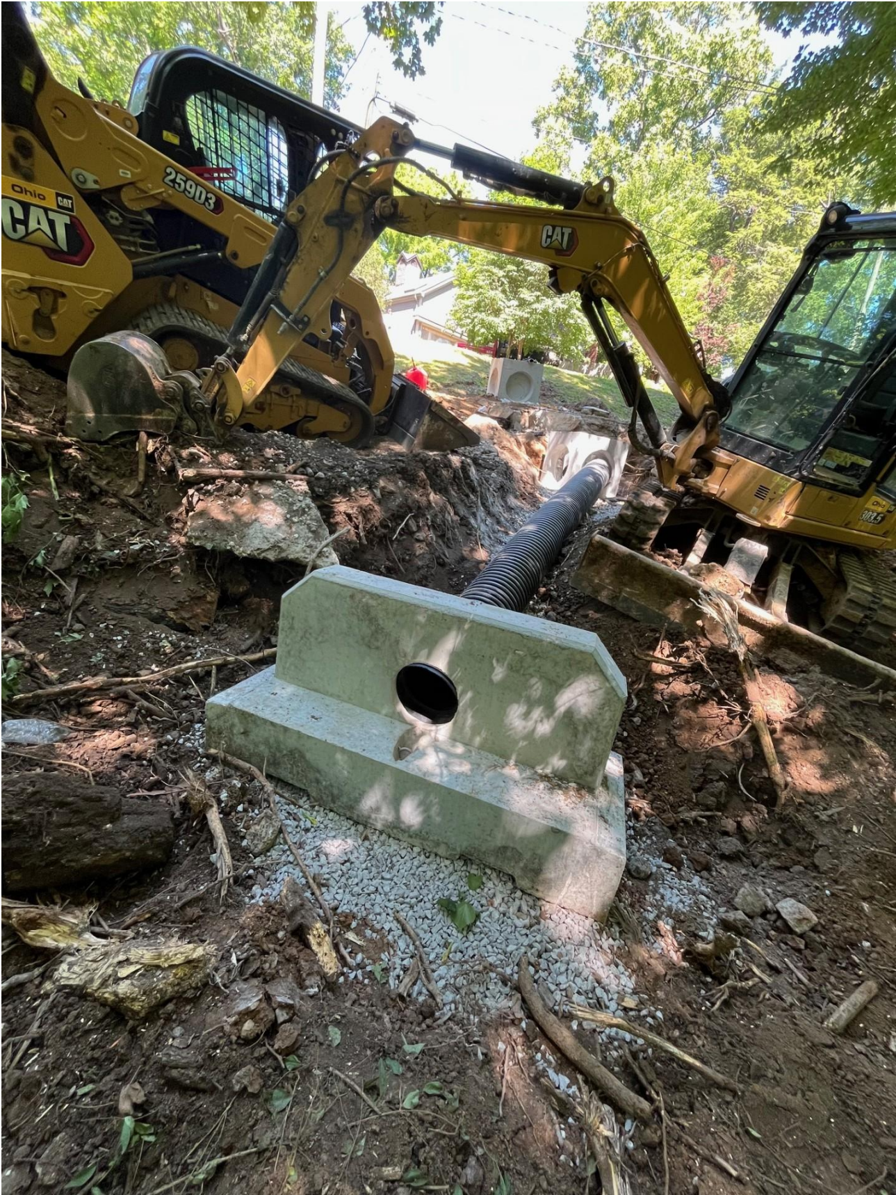
Images of erosion line and culvert installation at S. Ewing Ave.:
