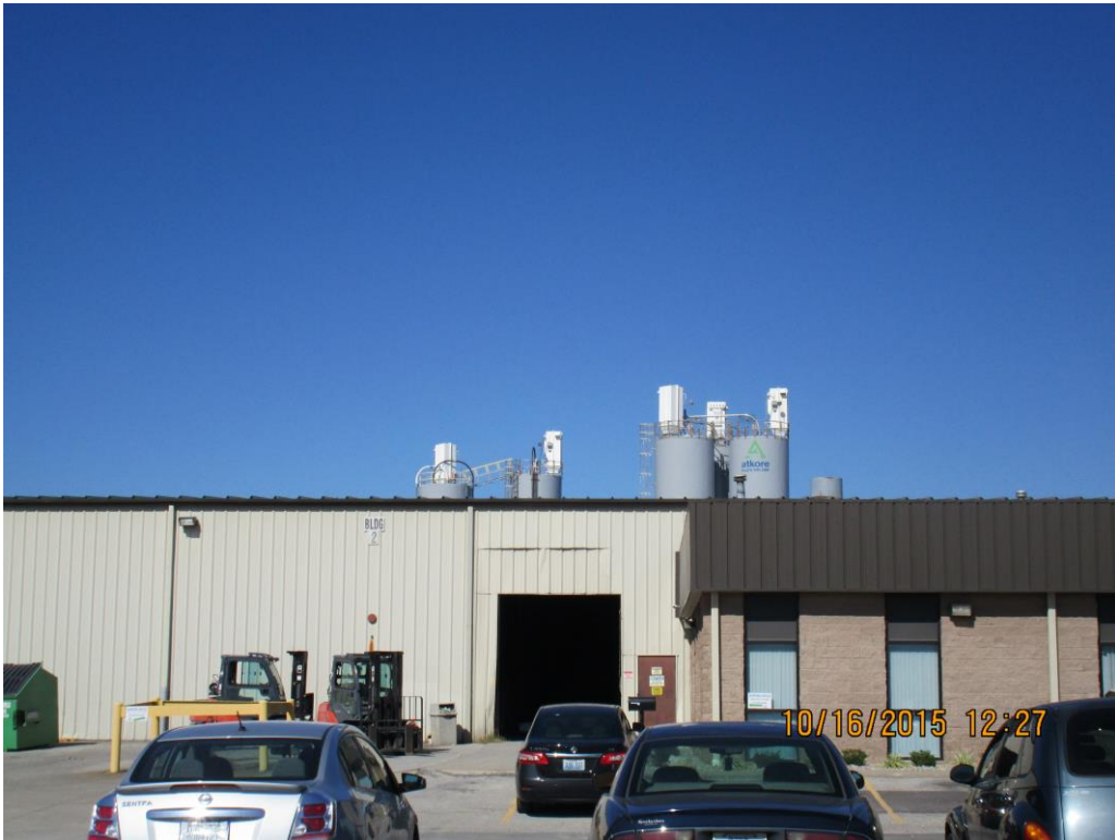
View from front of the building toward the rear and the location of the new addition
