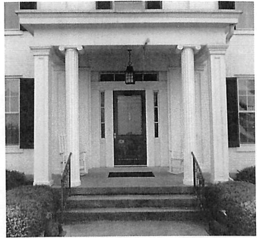
Single story porch with paneled posts and fluted Ionic columns at the James V. Harbison house.
