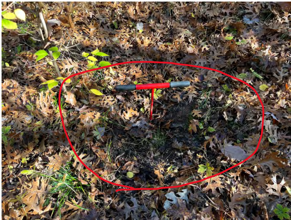
Photo 14: View of probe rod extended in partially closed throat located in F-17.
