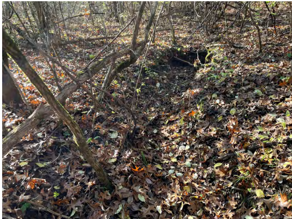
Photo 30: View of fan-shaped slope failure area SF-02.
