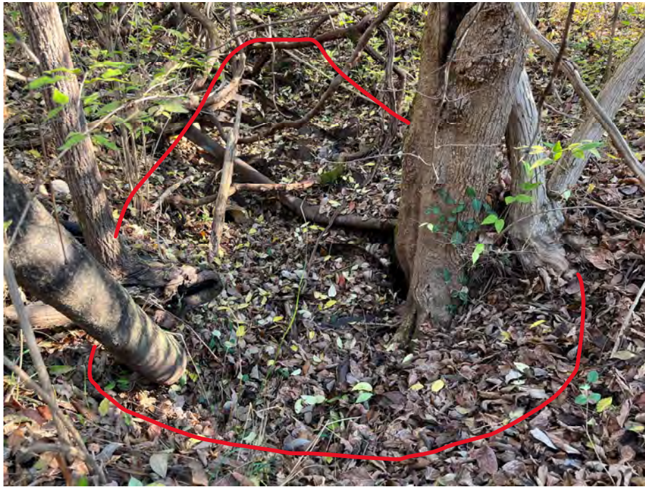
Photo 7: View of F-06 containing rusted debris and a partially closed throat.
