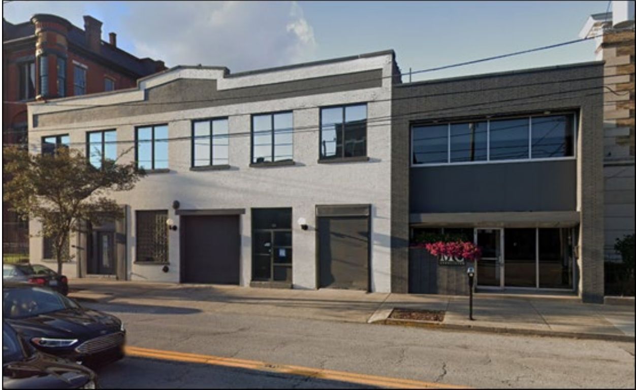
Building to be demolished, 625 E. Market - Google 2022
