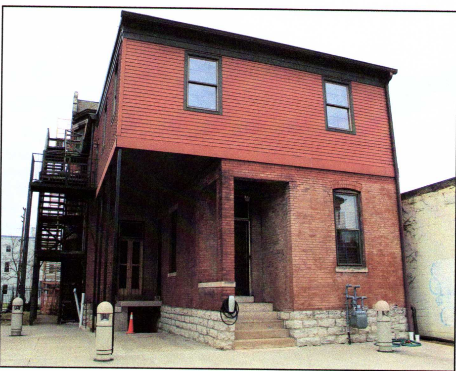
Rear facade facing the alley
