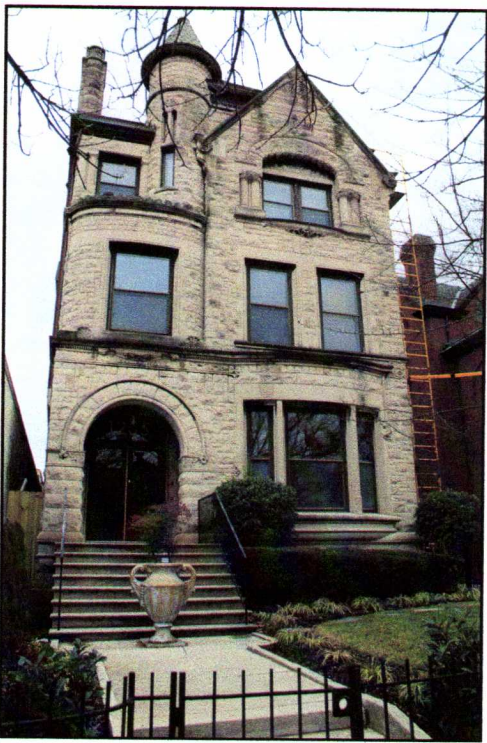
Front facade along S. 3rd Street
