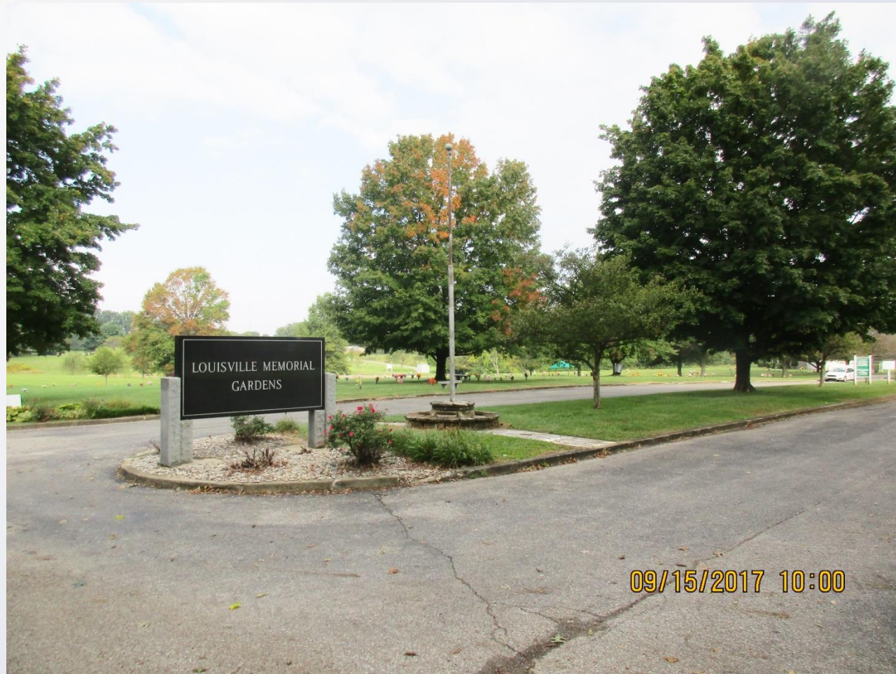
East Entrance Looking North to Roundabout
