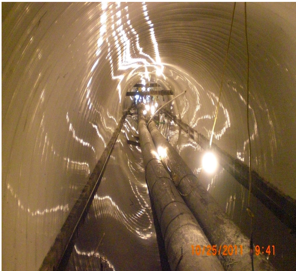
Above: Ohio River Interceptor
