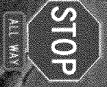
Remove Cross Traffic Does not stop. Replace Stop sign and install all-way Plaque
