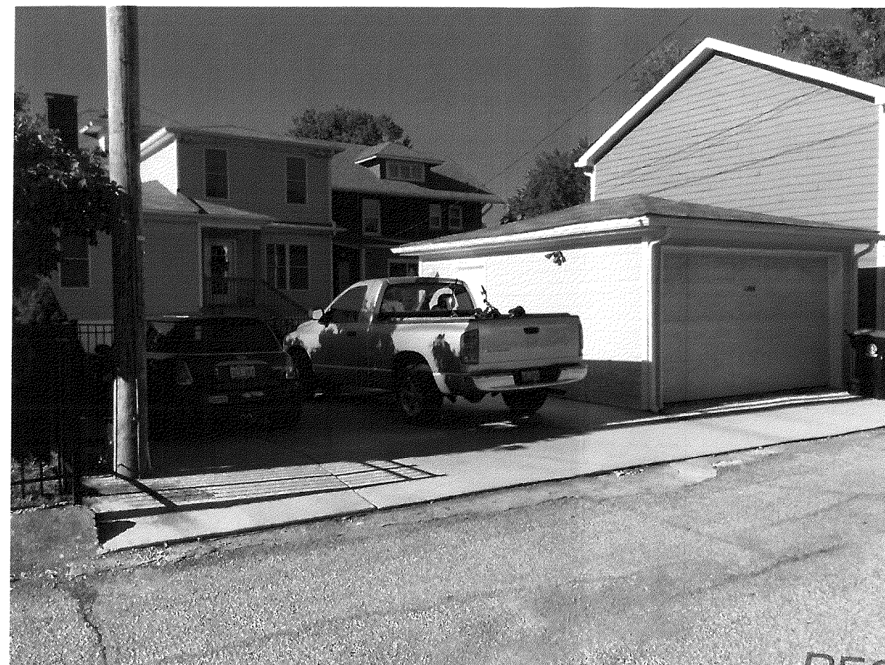
LOOKING NORTH FROM ALLEY
