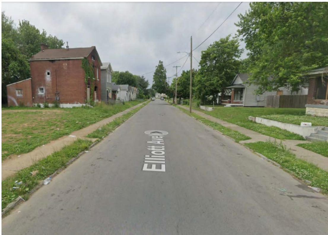
Images: College of Design School of Architecture at the University of Kentucky, Design Studio
