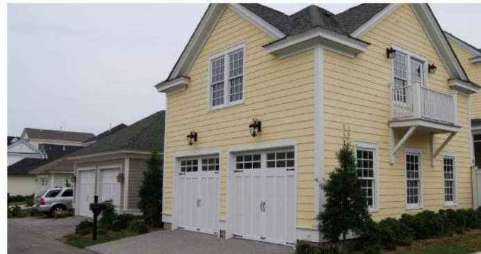
A Carriage House utilizes a large dormer to create a unit, over the garage.
