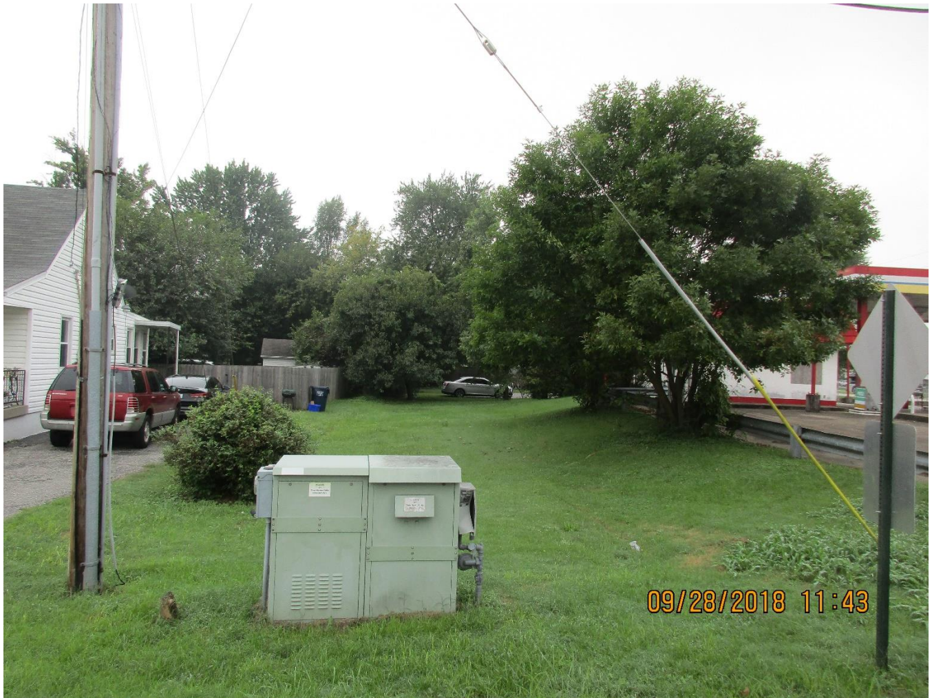
Area between the subject property and the property to the rear.
