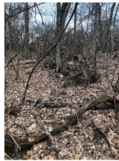
Steep slope in Area 3 where minor instability observed
