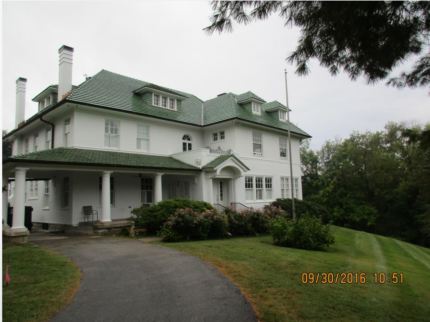
Looking southeast at the subject site.
