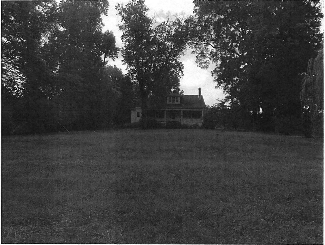
Looking south to the Powell-Smith House
