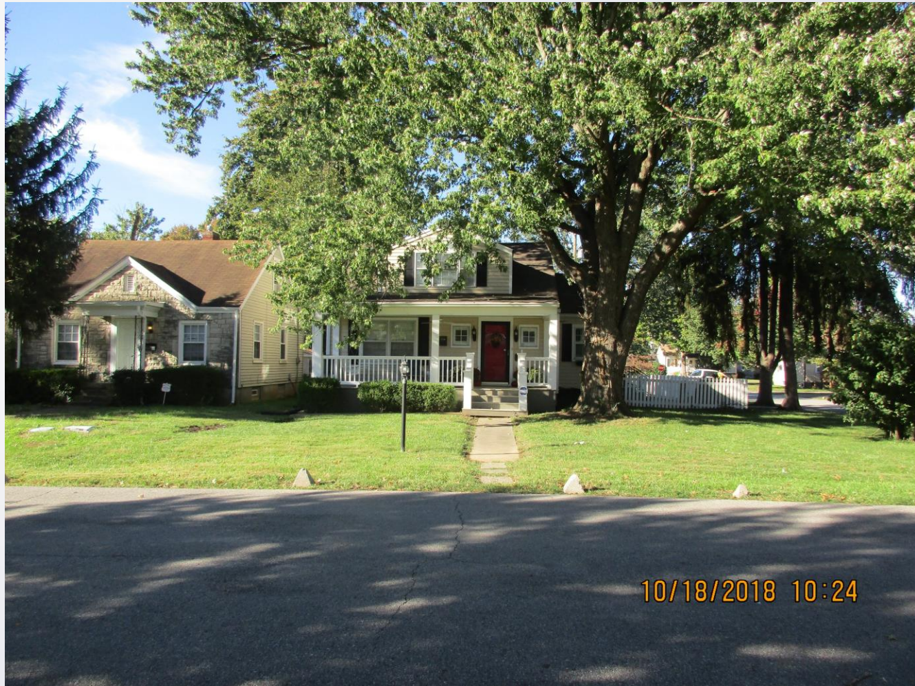
Property across Massie Avenue (left).
