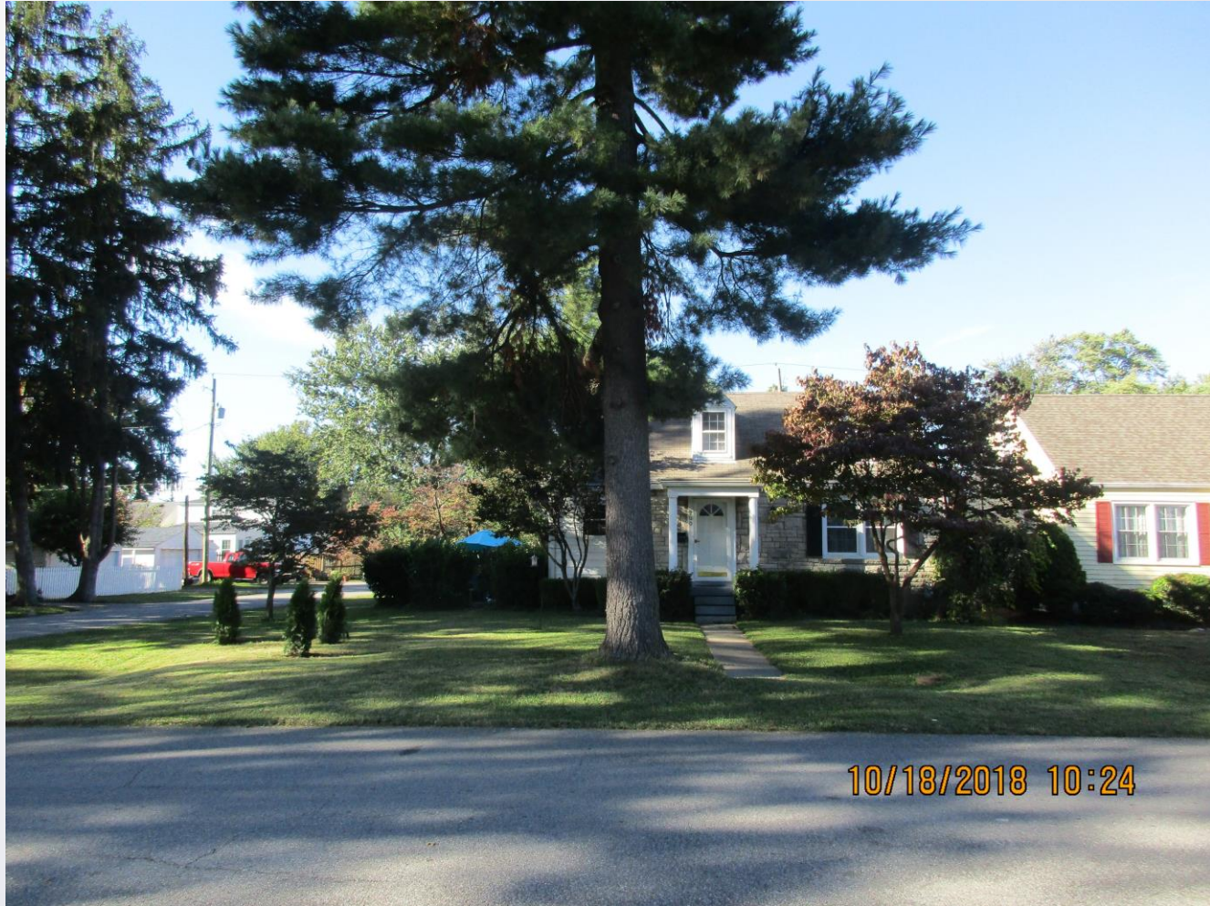
Front of subject property.
