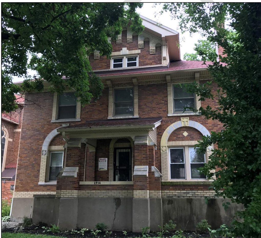
Figure 8. Front façade, or east elevation, of Building 2, the Rectory, looking west.
