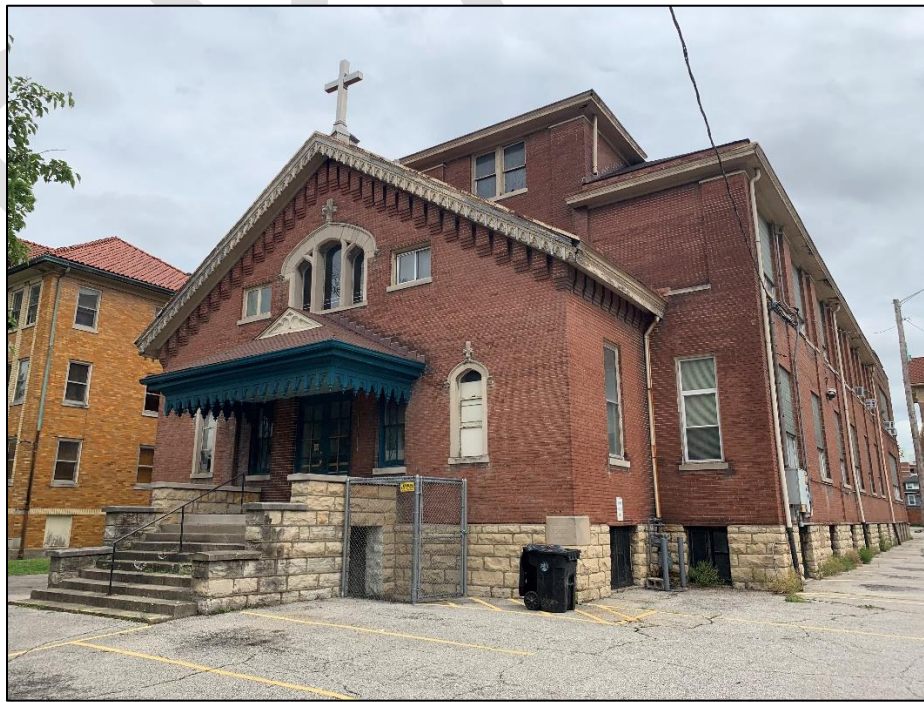
Figure 11. Front façade, or west elevation, of Building 3, the School, looking northeast.
