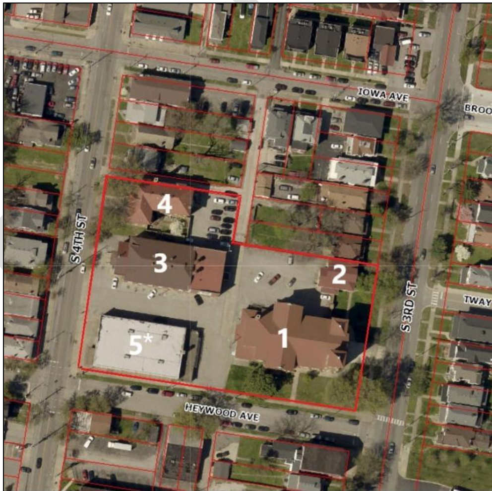
Figure 1. Aerial View of the Subject Property with a Building Key for Table 1 (LOJIC). *Building 5 is not included in this designation. This is not the designation boundary.
