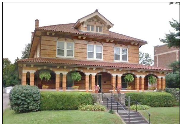
Figure 50. St. James Catholic Church Rectory, 1826 Edenside Avenue (Google)
