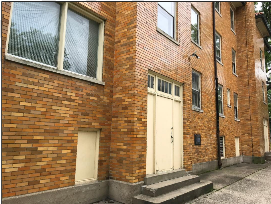
Figure 21. North elevation of Building 4, looking southwest.
