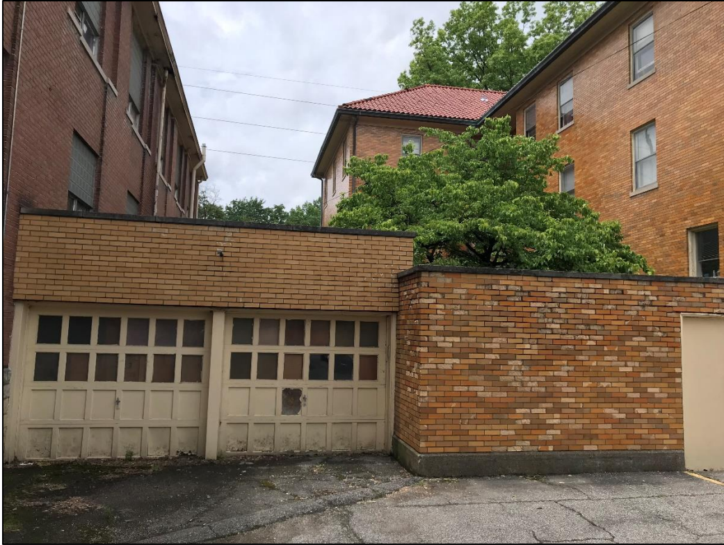
Figure 19. Garage and courtyard wall connecting Building 3 and Building 4, looking west.
