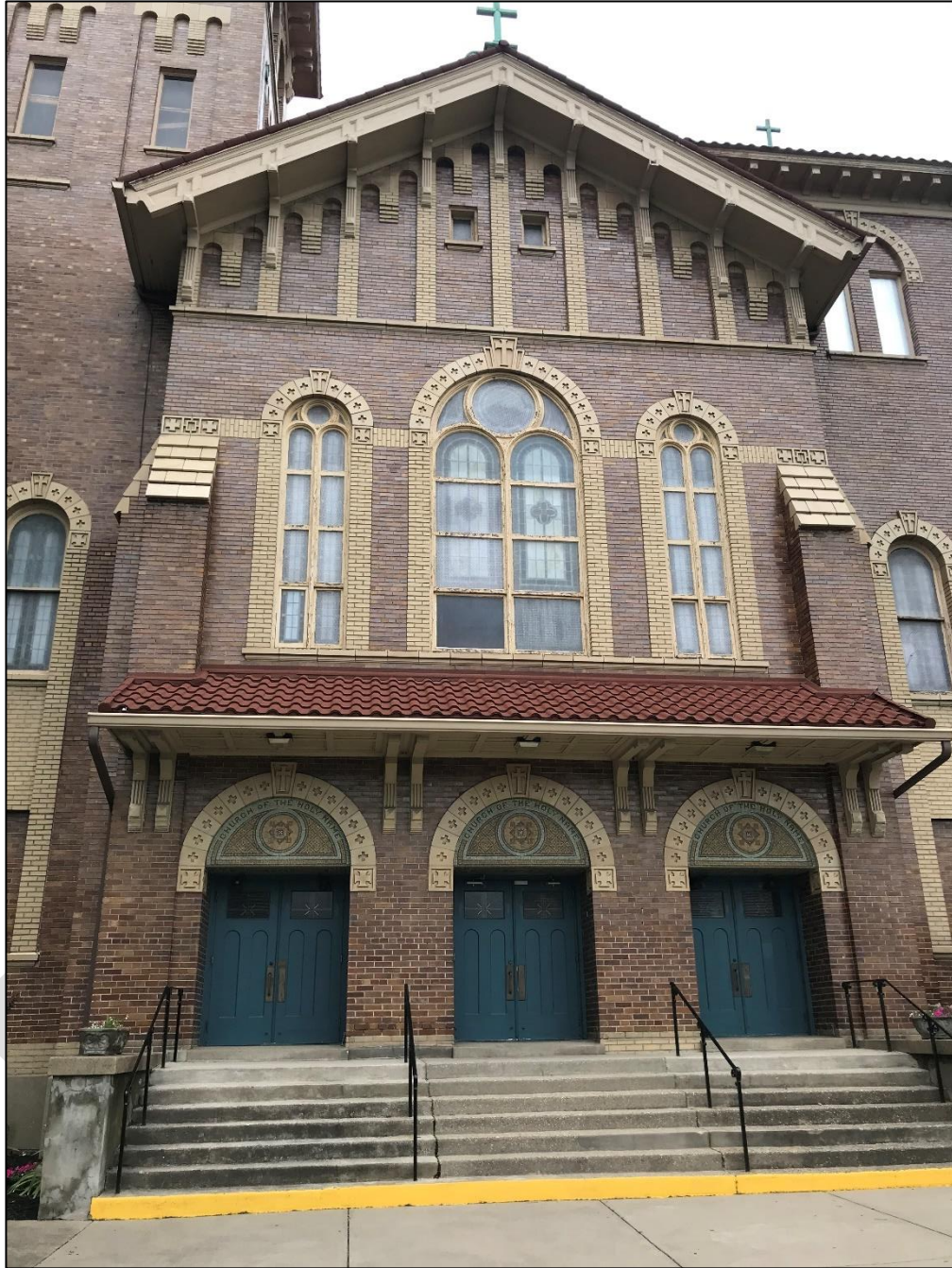
Figure 3. Front façade detail of the gable section of Building 1, looking west.
