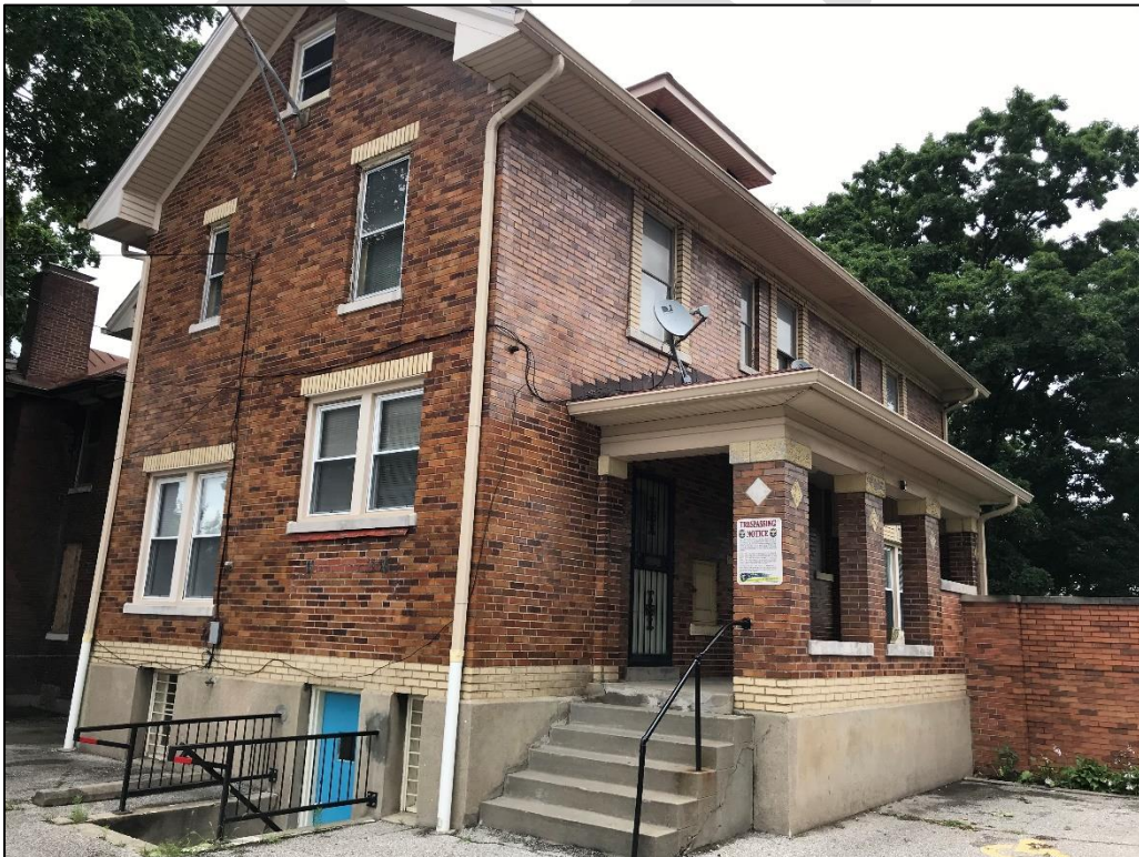
Figure 10. West and south elevations of Building 2, looking northeast.
