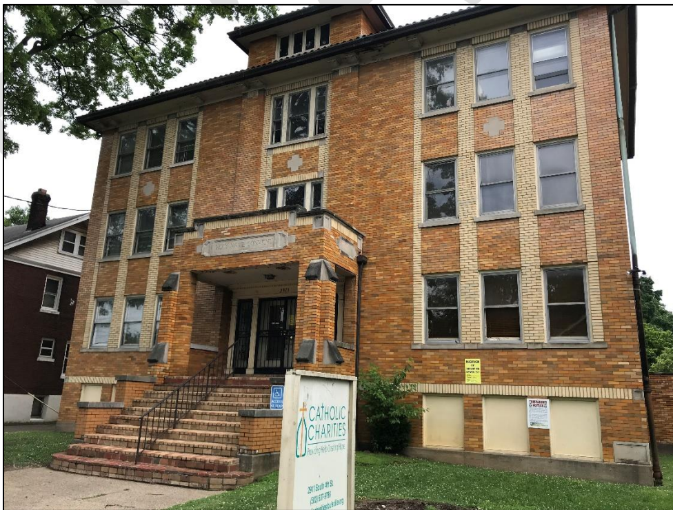
Figure 15. Front façade, or west elevation, of Building 4, the Convent, looking east.
