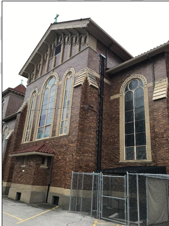
Figure 5. North elevation of Building 1, looking southeast.
