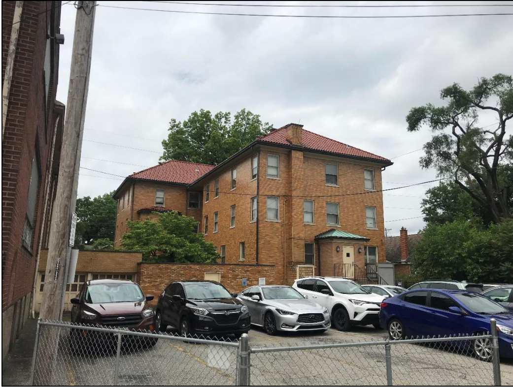
Figure 17. South and east elevations of Building 4, looking west.
