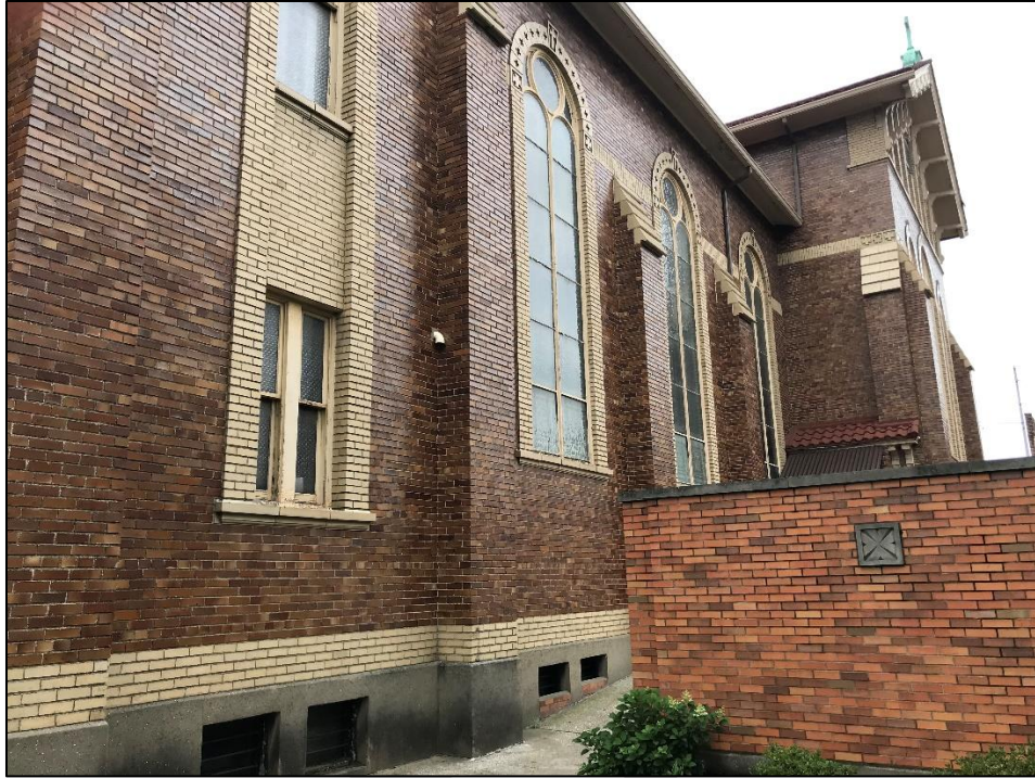
Figure 4. North elevation of Building 1, looking southwest.
