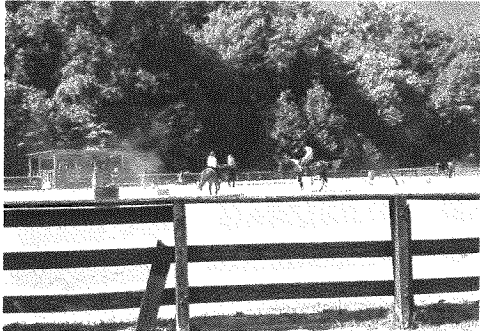
Missing and broken boards
