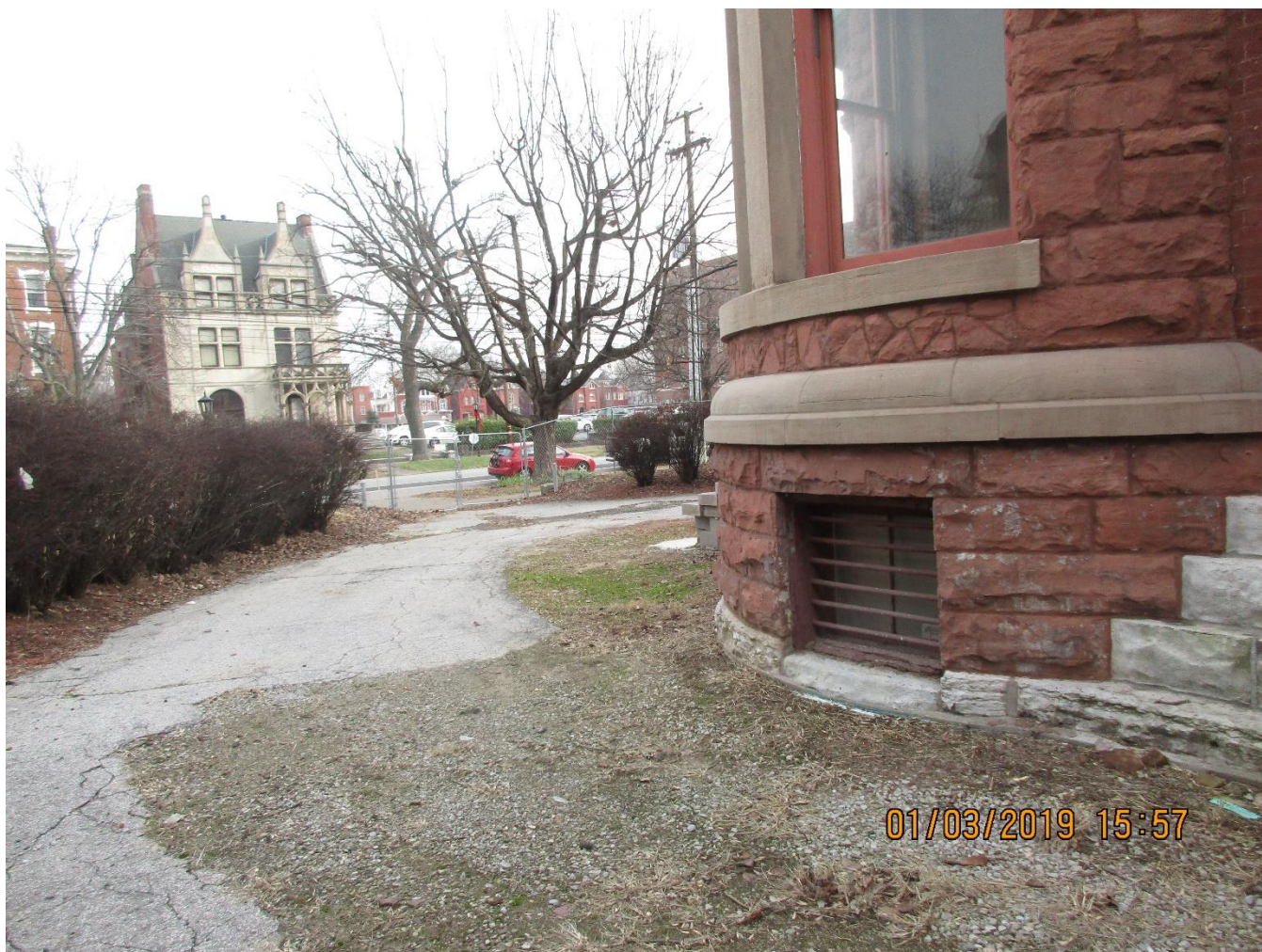
Existing access from 3 rd Street.
