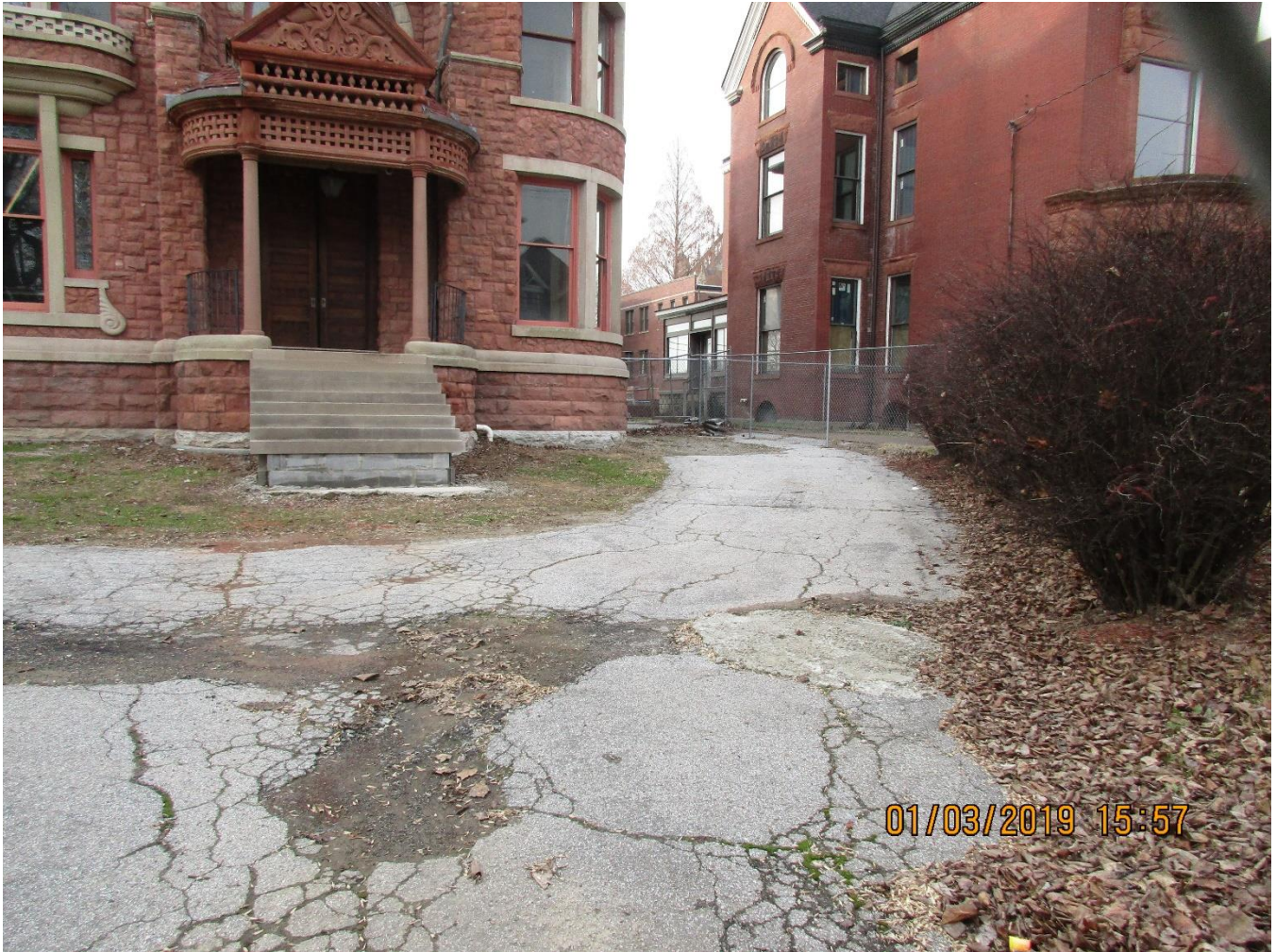
Existing access from 3 rd Street.
