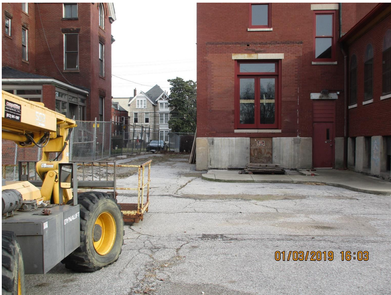
Location of proposed dining room expansion and access from 3 rd Street.
