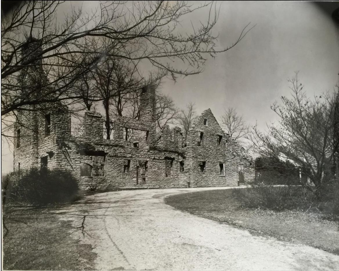
Image 12. Southwest and southeast elevation of 609 Blankenbaker Lane, circa 1951 (courtesy Filson Historical Society, Stratton Hammon Photograph Collection).
