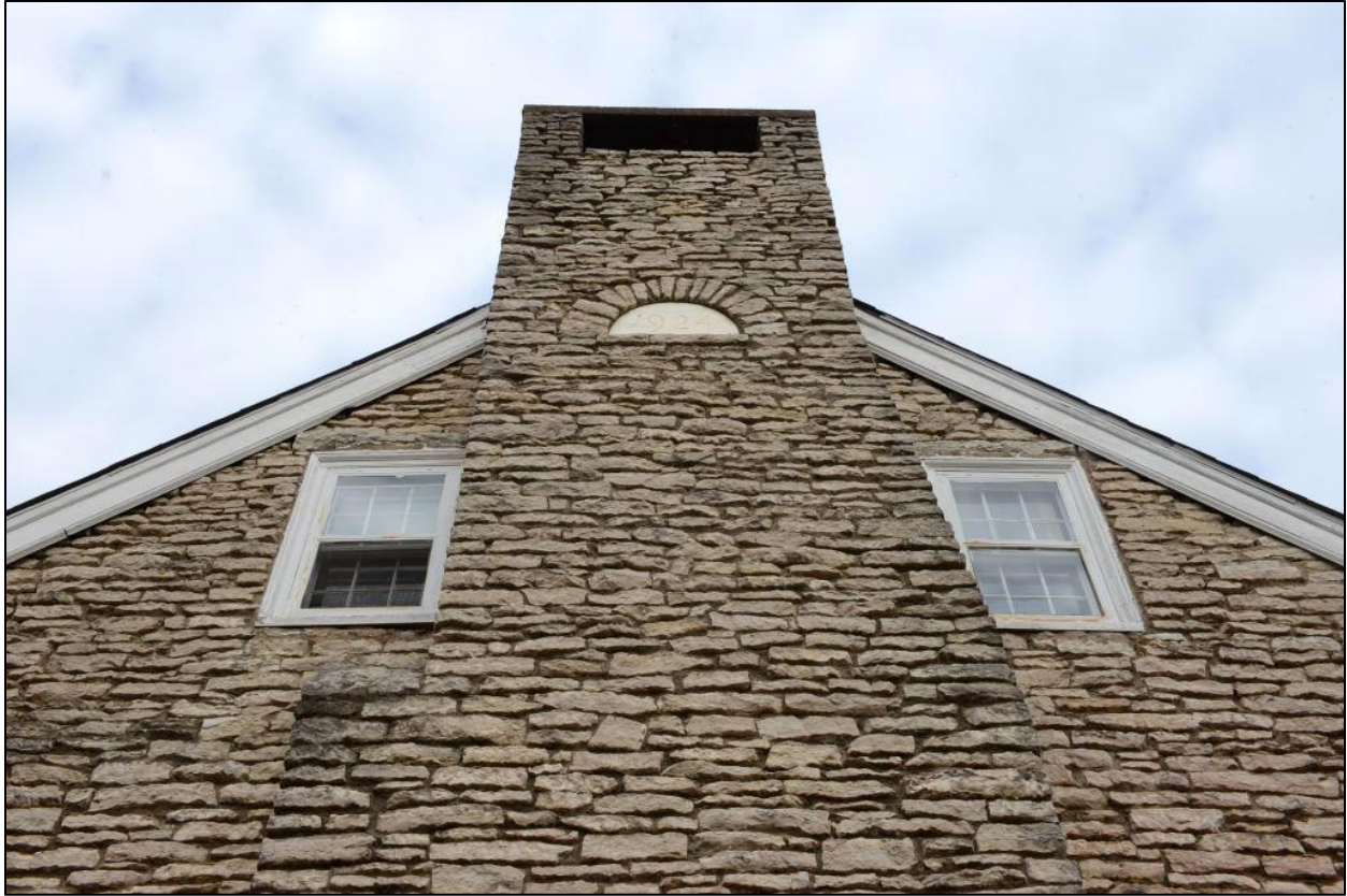
Image 10. Chimney detail, southwest elevation of 609 Blankenbaker Lane.
