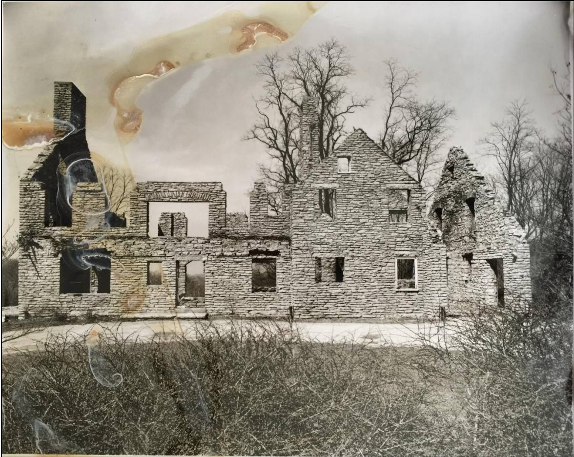
Image 13. Southeast, rear, elevation of 609 Blankenbaker Lane, circa 1951 (courtesy Filson Historical Society, Stratton Hammon Photograph Collection).
