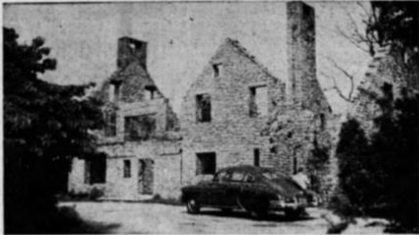
These gaunt stone walls and chimneys were all that was left of the home of Dr. John Walker Moore on a hill overlooking Blankenbaker Lane after fire swept it in 1930.
