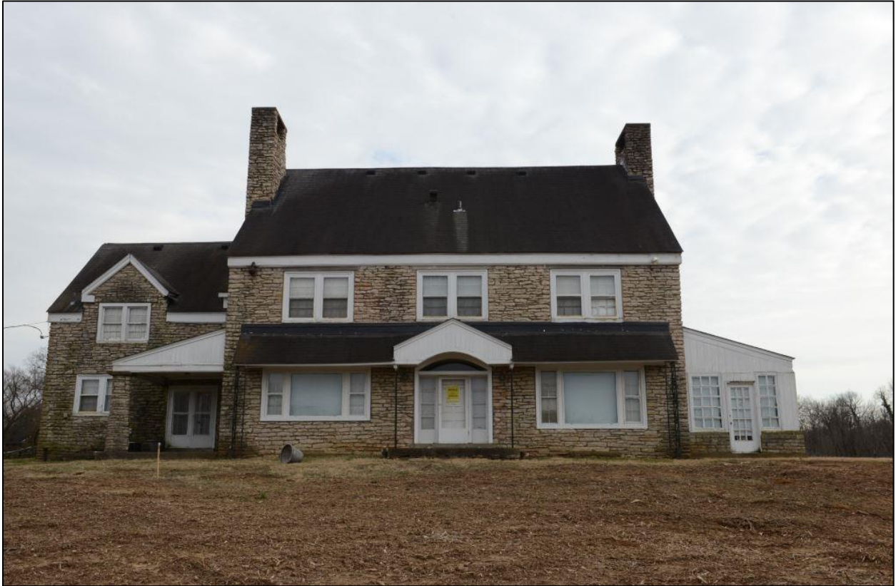
Image 6. Northwest, front, elevation of 609 Blankenbaker Lane.
