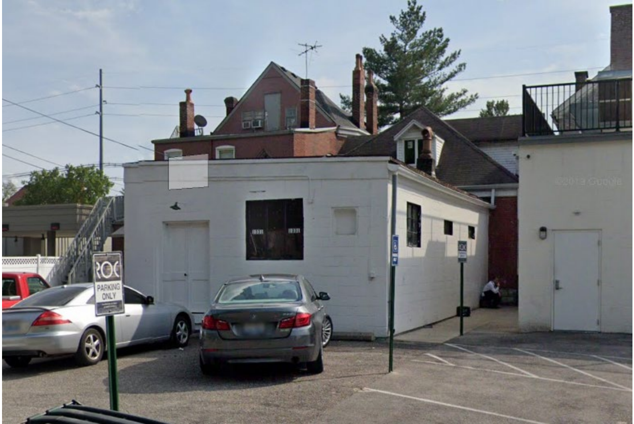
1331 Bardstown Rd. Rear - Google May 2019
