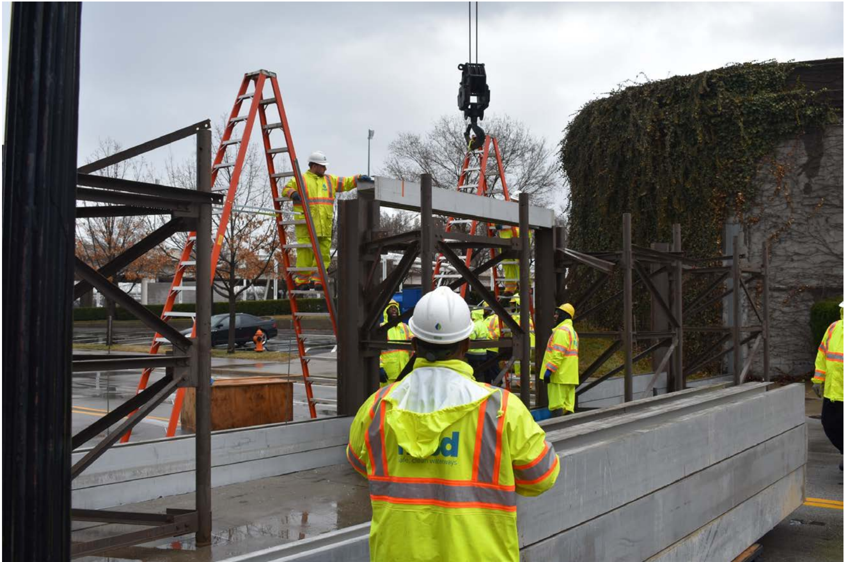
Bingham Way Street Closure
