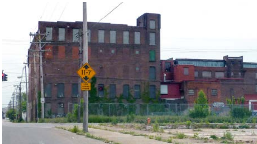
Current and former industrial uses cluster around the two rail lines
