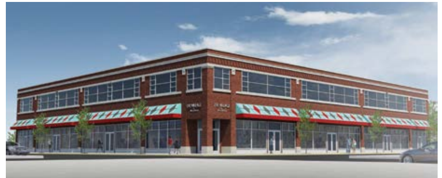
Rendering of MOLO's "The Village at West Jefferson" at the corner of 12th Street and West Jefferson. Photo courtesy of Molo Village CDC.
