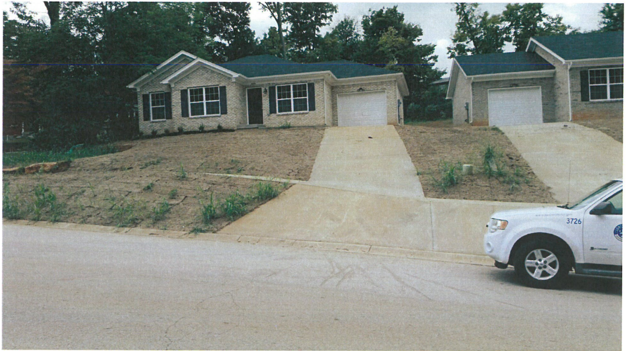
6209 Whispering Hills Blvd - Current condition, most cars cannot mount driveway, bottom-out at sidewalk
