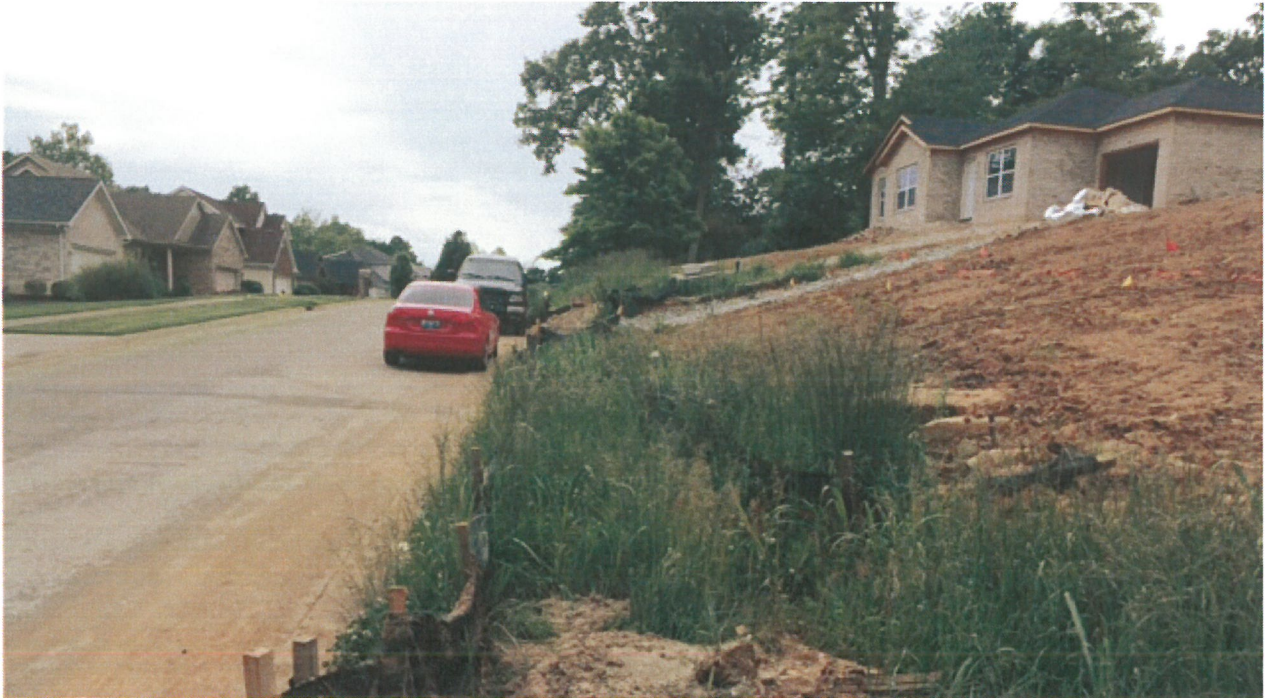
West on Whispering Hills Blvd., site on the right. Sidewalk provided on other side of road.
