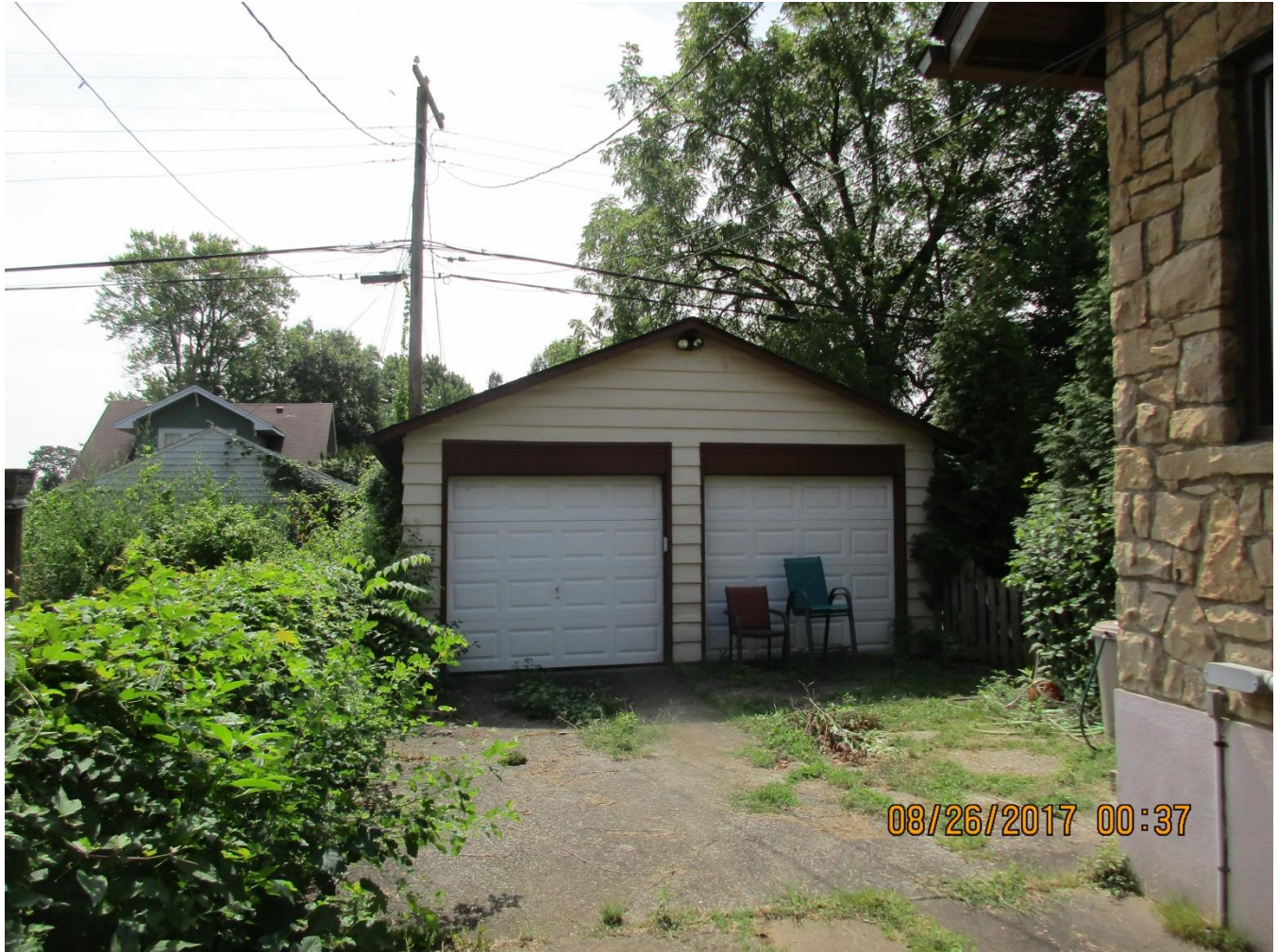
The garage which is to be remodeled.
