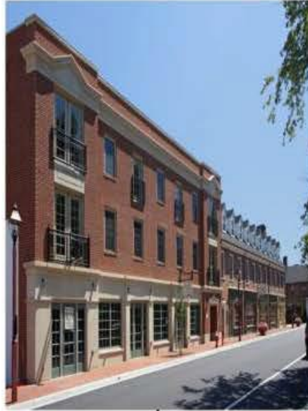
CAST STONE RETAIL LEVEL AND BRICK ABOVE
