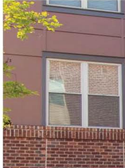
TRANSITION FROM BRICK TO BOARD AND BATTEN
