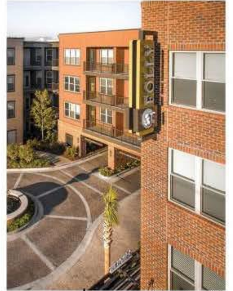
PARKING ENTRANCE and BALCONY DETAIL
