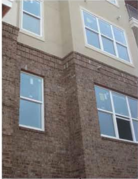
TRANSITION OF BRICK TO BOARD BATTEN
