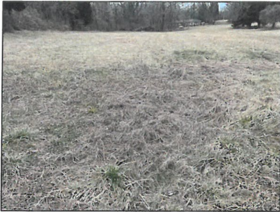
PHOTO NO. 7: Ground subsidence/differing vegetation (Feature 5)
