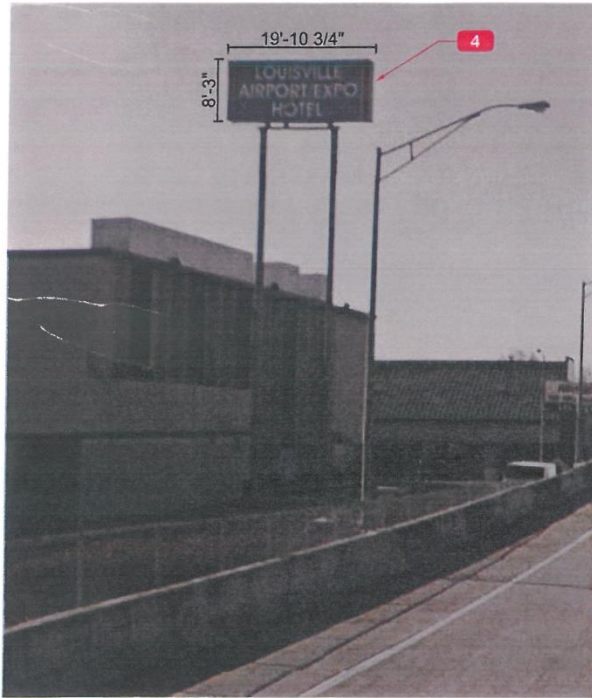
Existing Double-Faced Internally Illuminated Hi-Rise Sign
