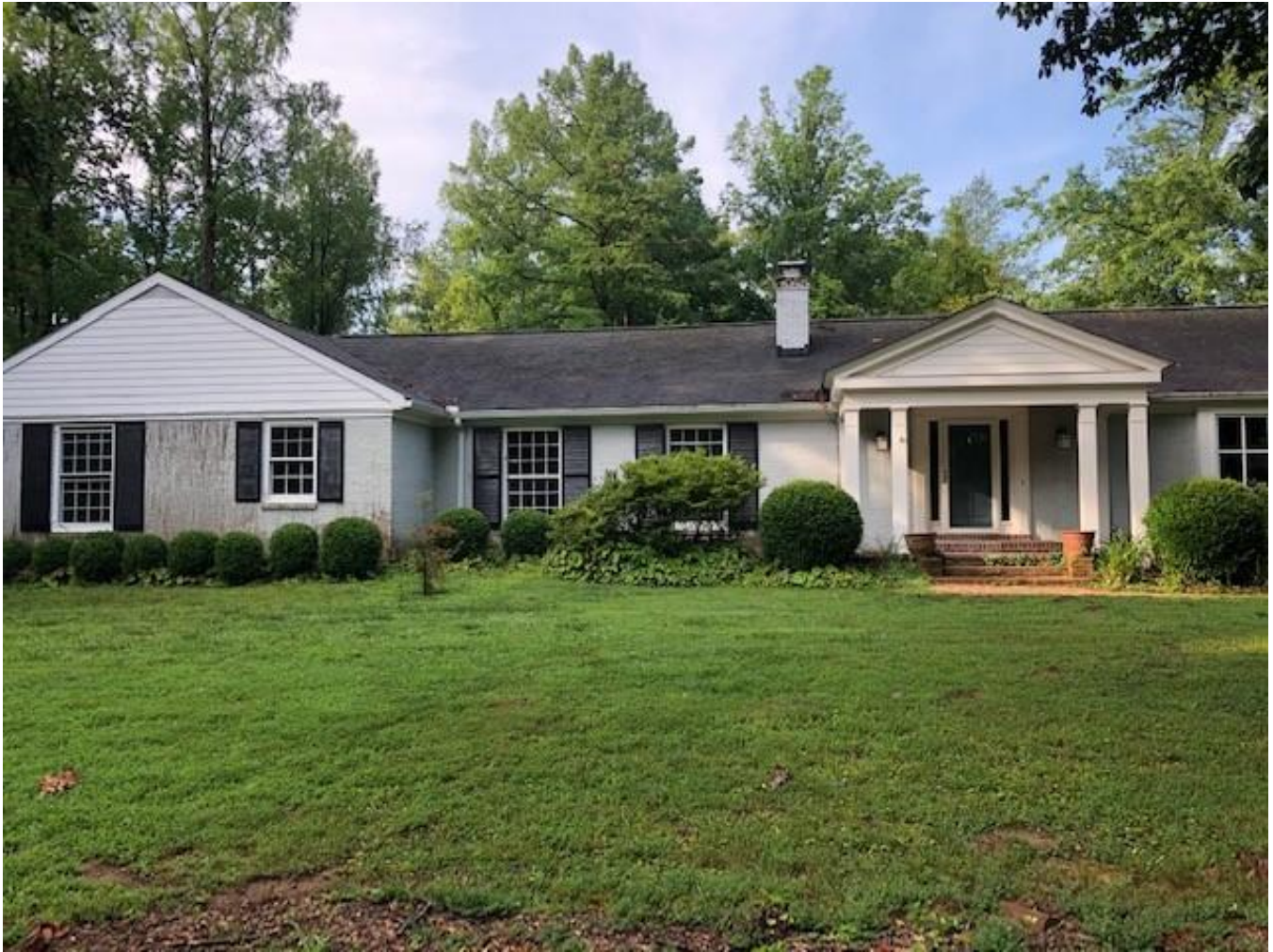
Front of subject property and location of proposed addition.
