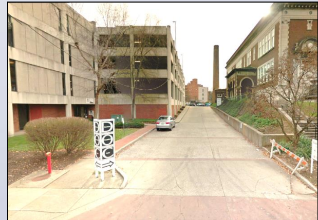
West property line with garage at rear
