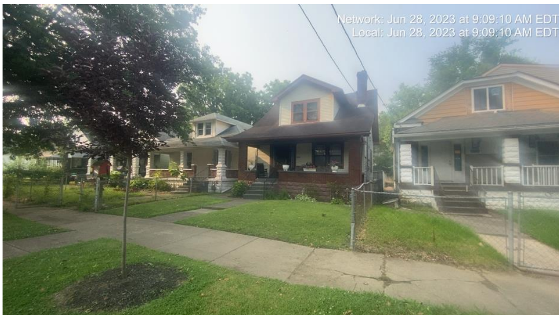
Left of subject site.
