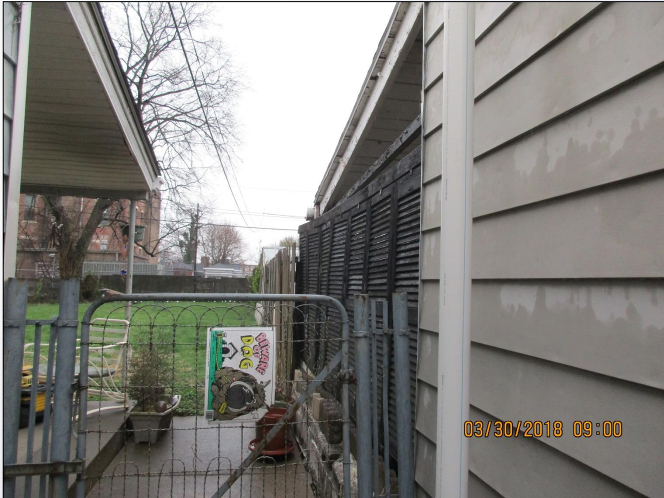
The separation between existing structures.
