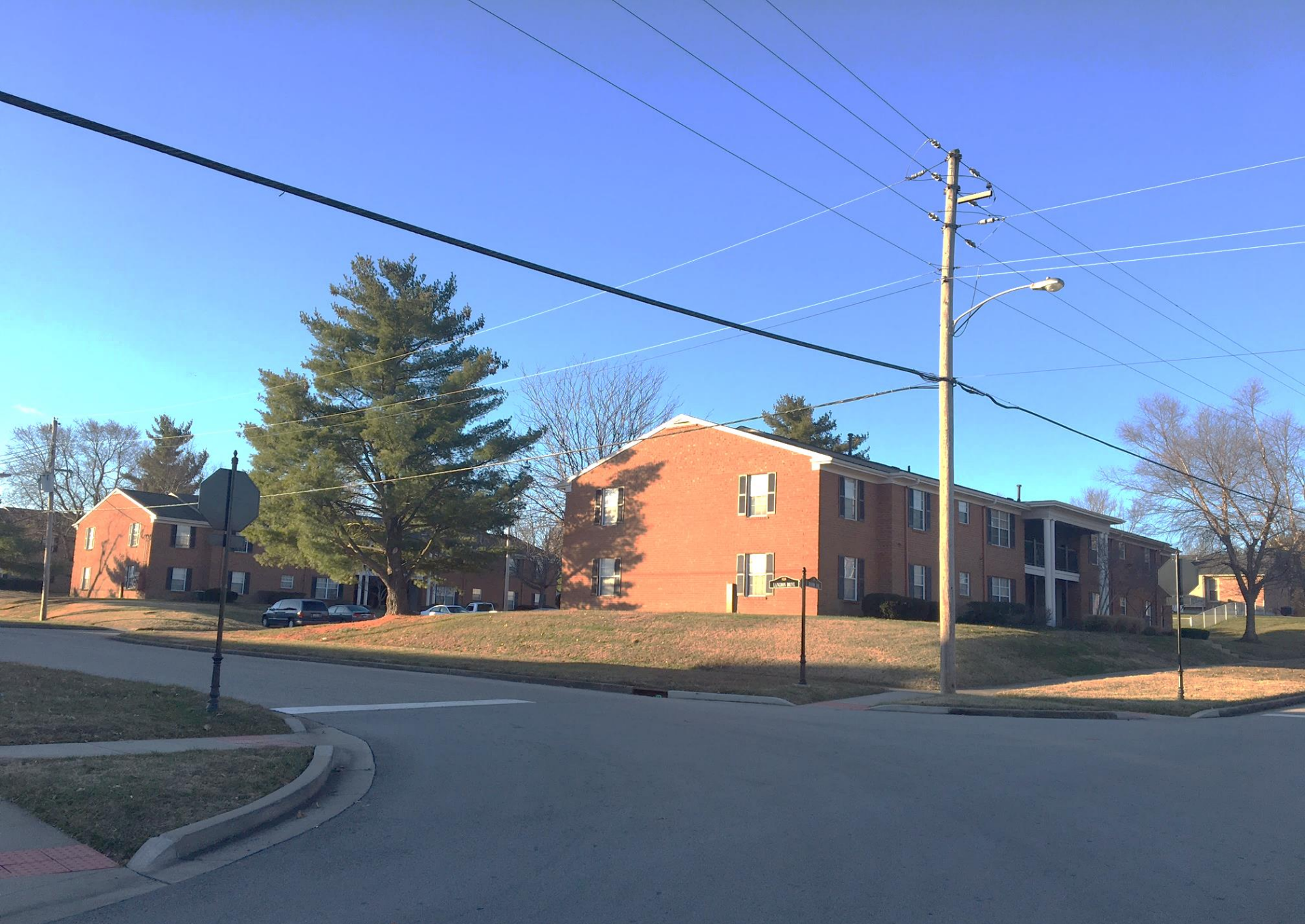
Blossom Lane and Langdon Drive – southwest of site
