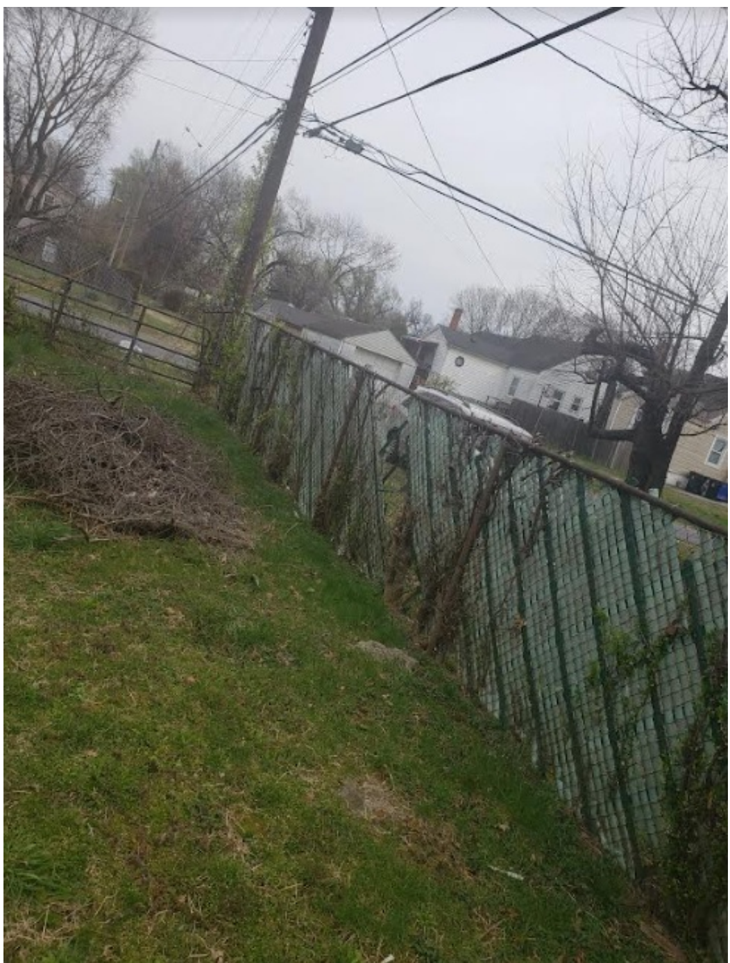
THE OWNER IS PROPOSING TO REPLACE THIS 6' FENCE
