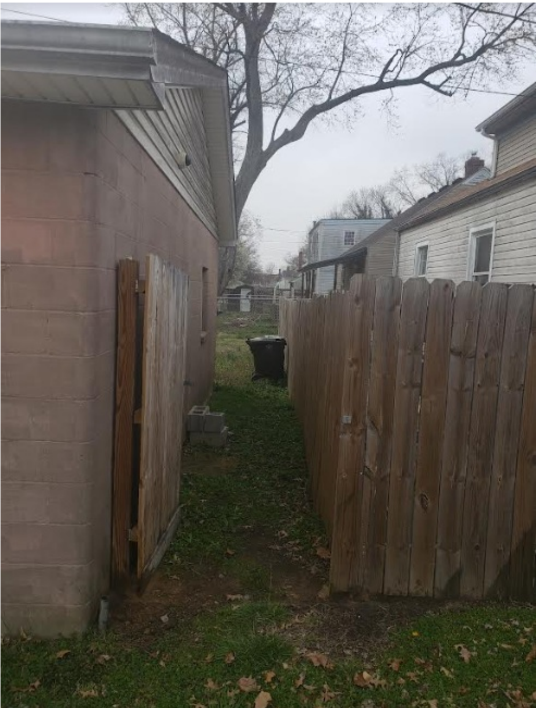
SHOWING THE DISTANCE BETWEEN THE EXISTING ONE-STORY GARAGE AND THE EXISTING BACK OF HOUSE
