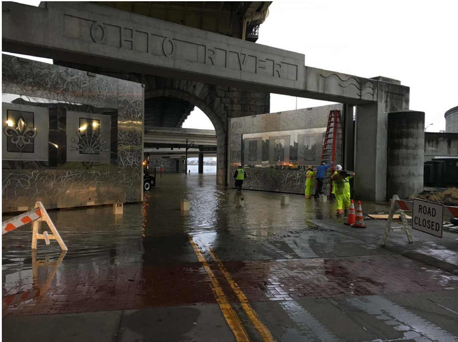
2 nd Street Swing Gate Closure
