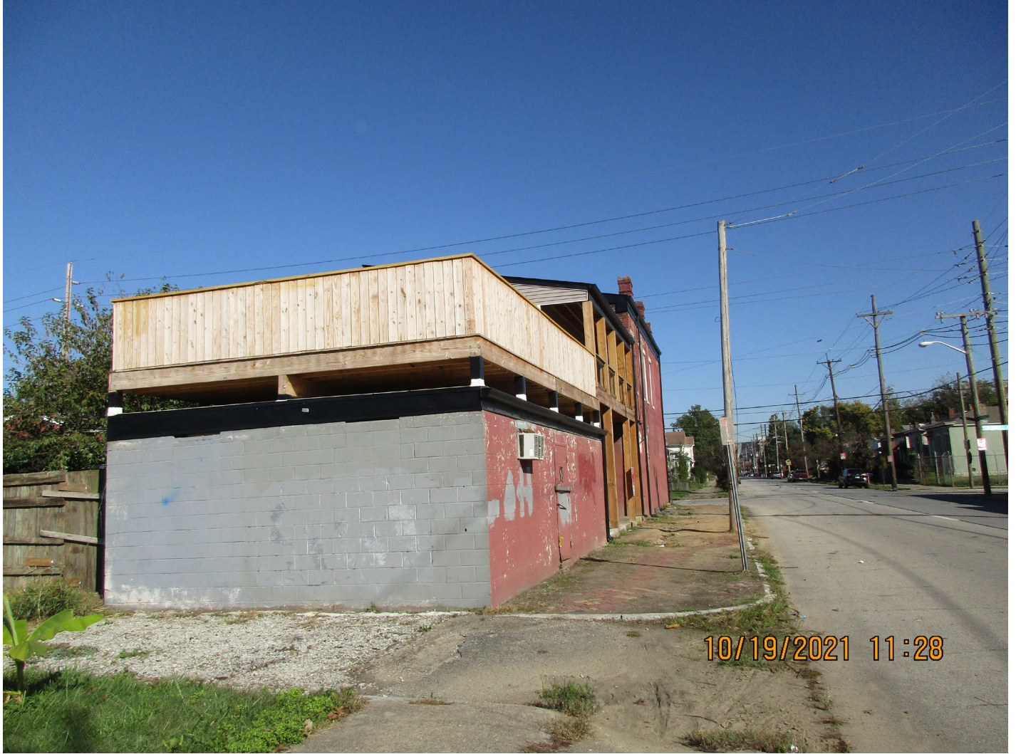
View of variance area along S. Jackson St. from rear of property.
