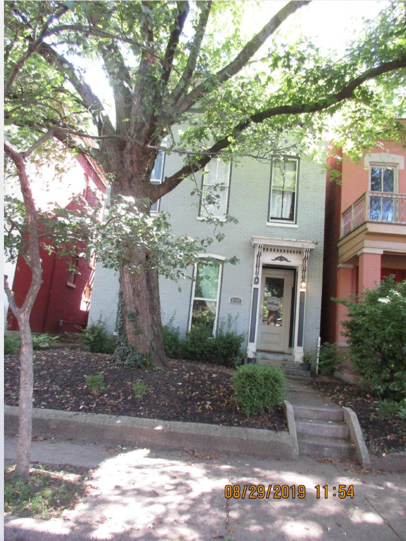
The front of subject property.
