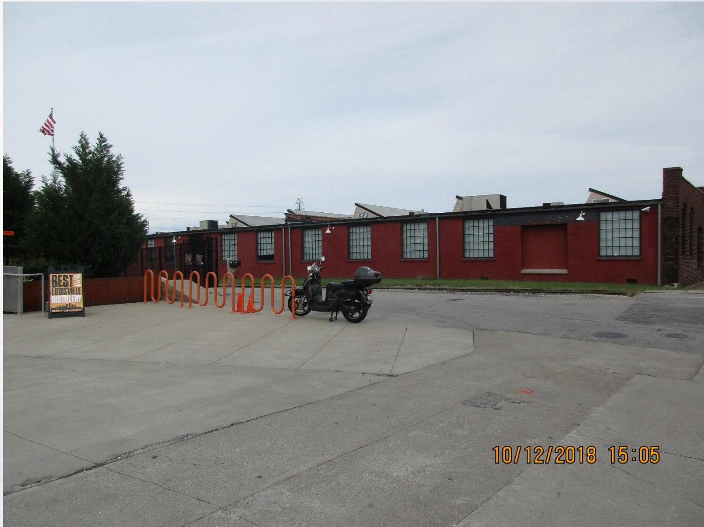
Adjoining Property to East
