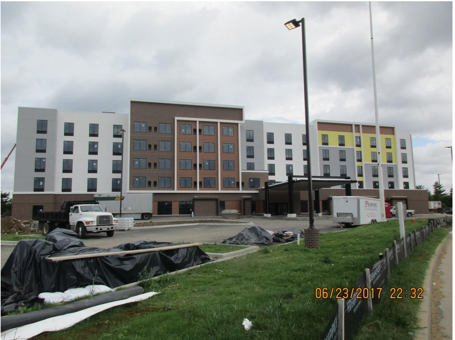
The south elevation of the hotel under construction.
