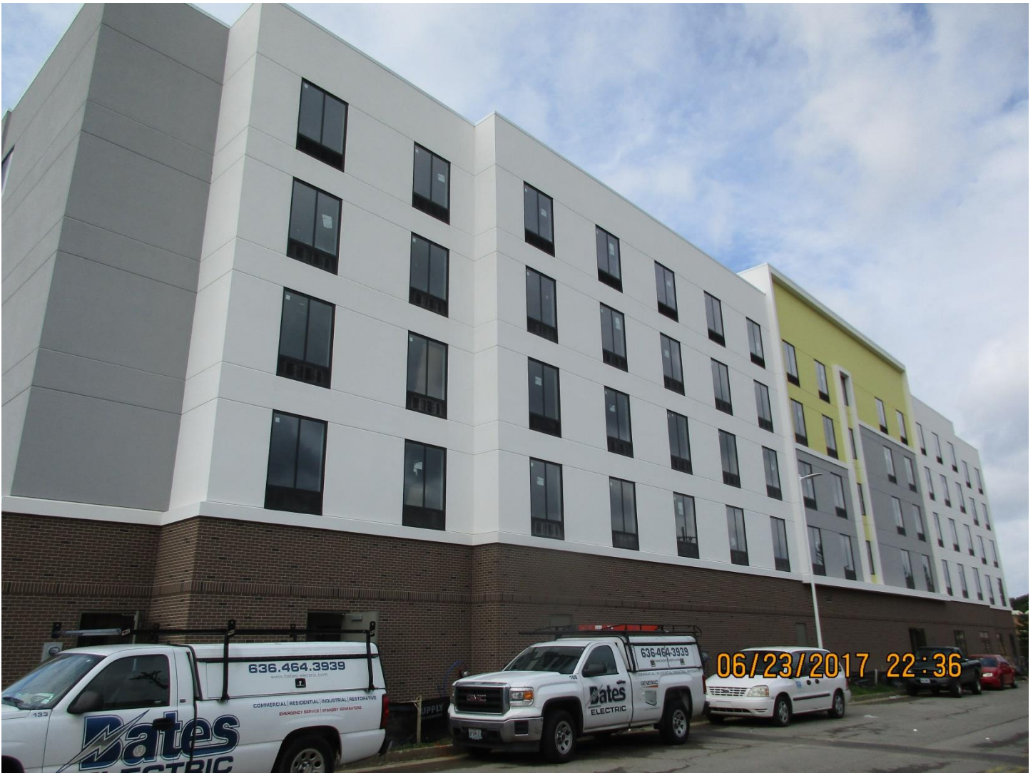
The north elevation of the hotel under construction.
