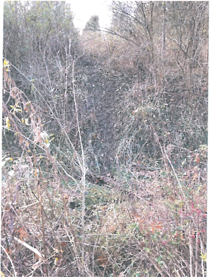
Steep stream bank at Area 01
