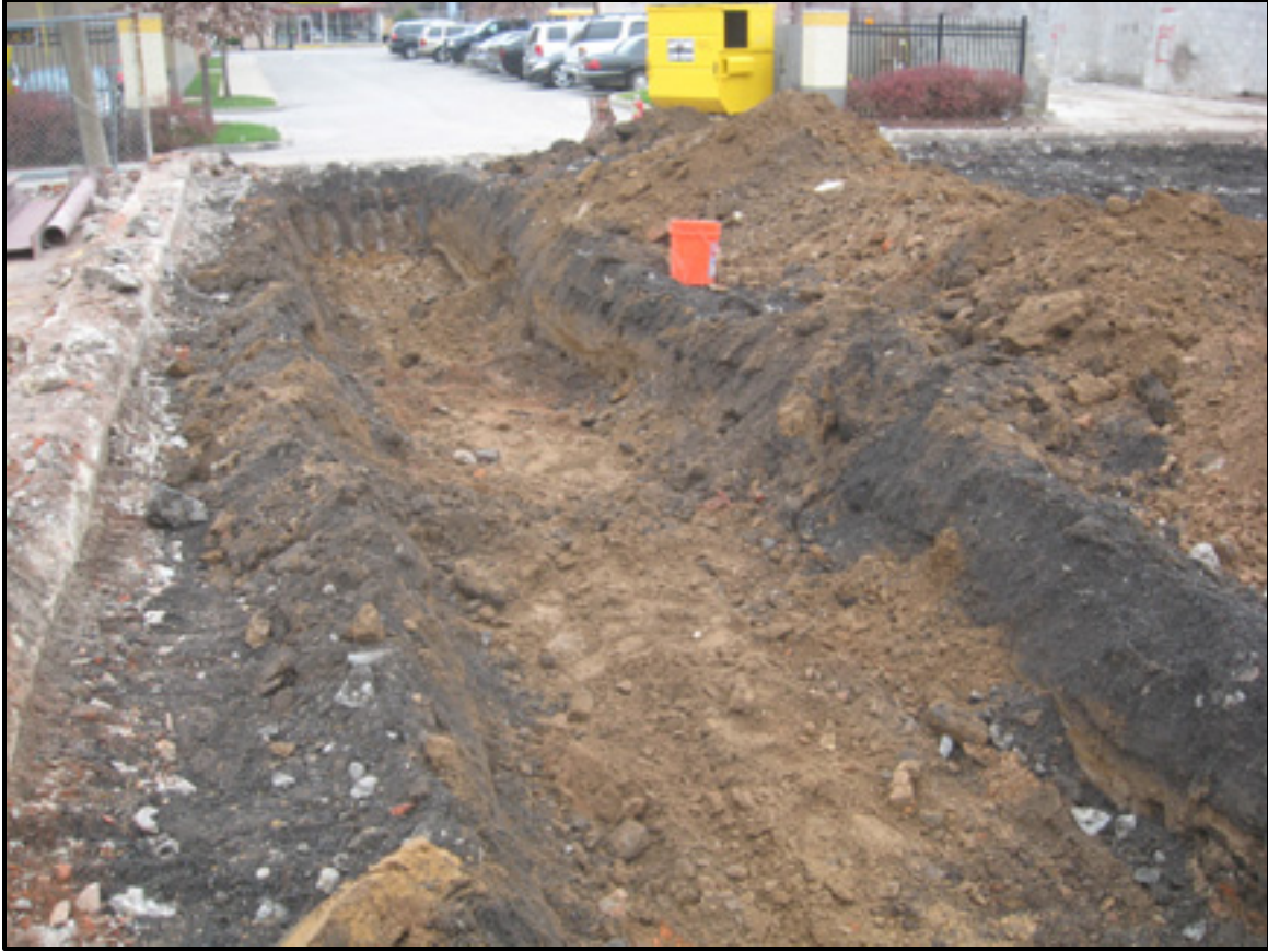
Figure 2-12. Photograph of the Test Trench Excavated in 2009.
