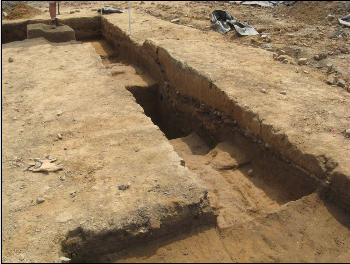
Figure 5-6. Photograph of the West Wall Profile Looking Southwest.
