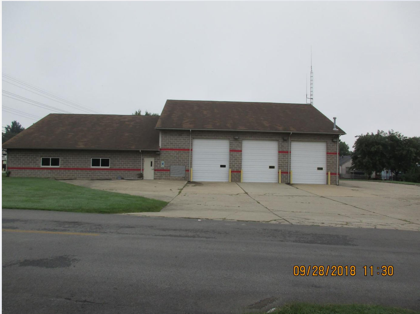
Property across Luken Drive from the subject property.
