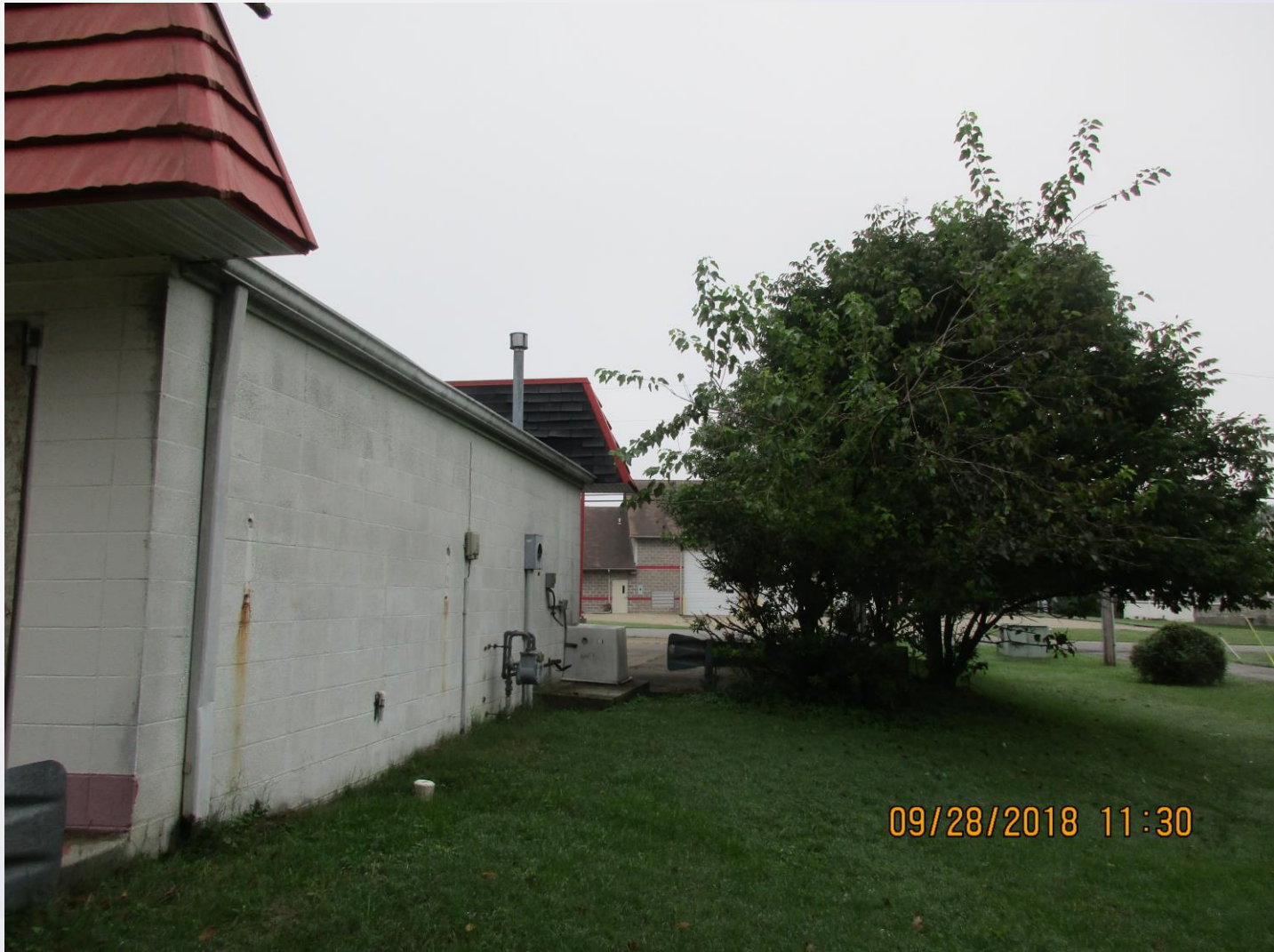
Rear of existing building.
