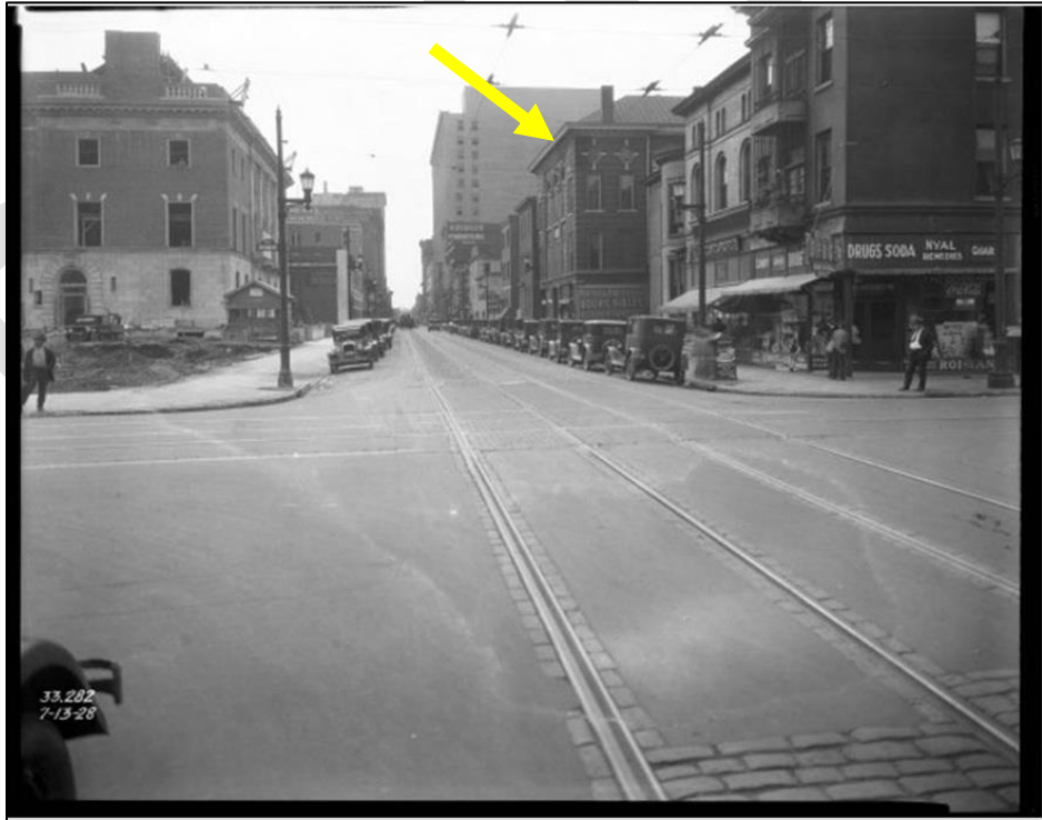
Figure 18. Photo of View looking west at the intersection of W. Walnut St. and S. Second St. Liberty Hall is visible in the center of the photo.
