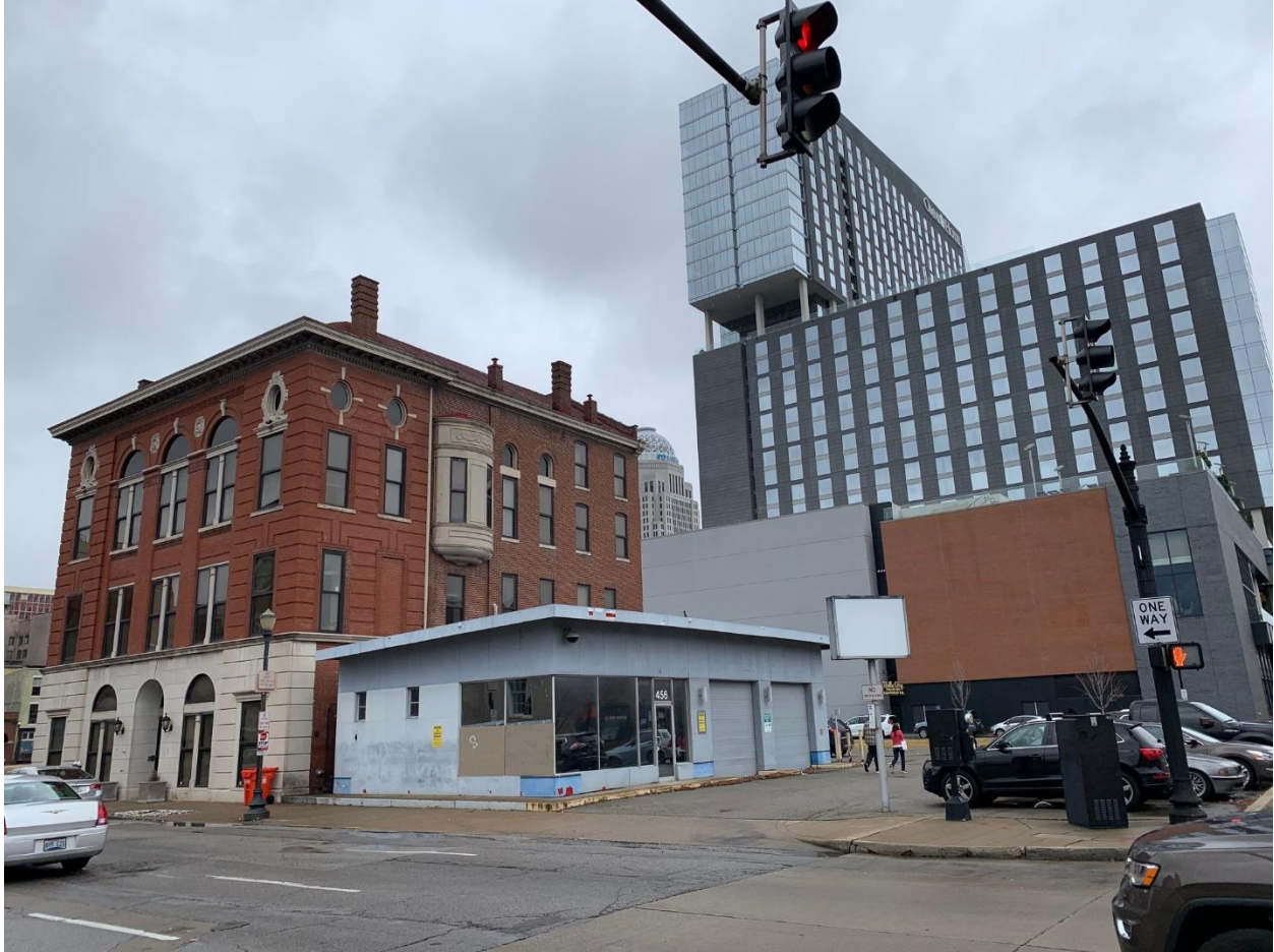
Figure 12. Current day view looking at northwest at the East and South elevations at the corner of S. Second St. and W. Muhammad Ali Blvd. (formerly W. Walnut St.).
