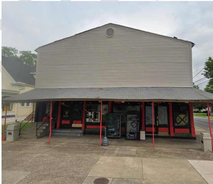
Figure 24. Klondike Hall, 2201 Garland Ave.
