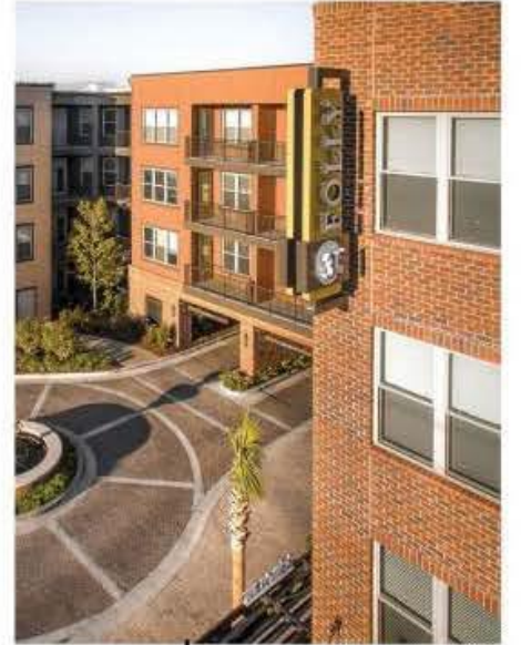
PARKING ENTRANCE and BALCONY DETAIL
