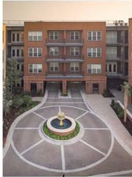
BRICK DETAIL and PARKING ENTRANCE
