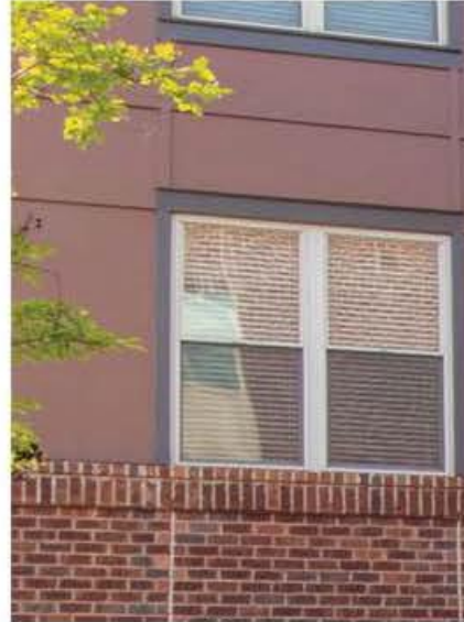
TRANSITION FROM BRICK TO BOARD AND BATTEN
