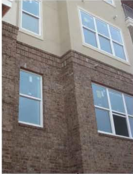
TRANSITION OF BRICK TO BOARD BATTEN
