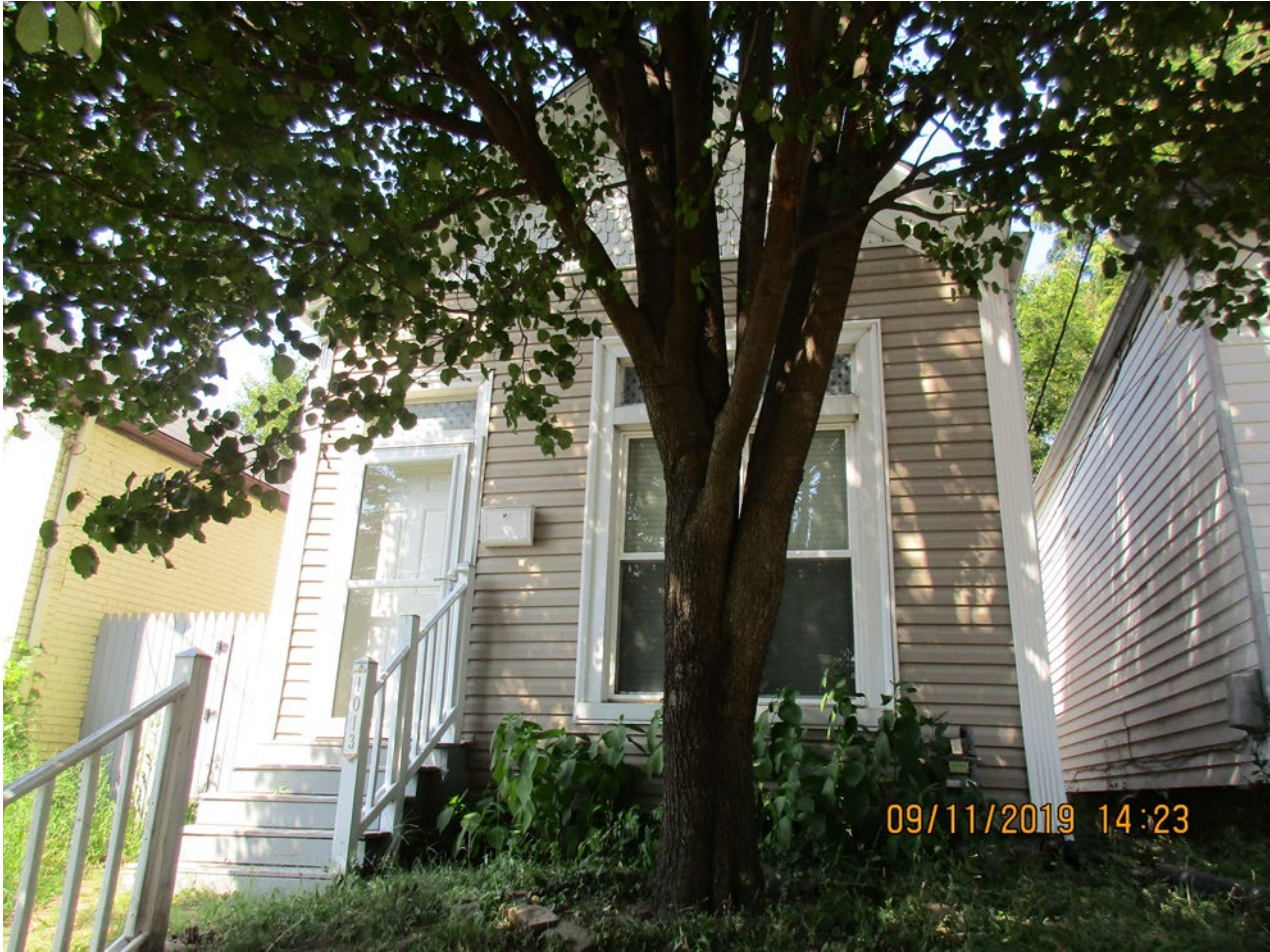
Property to the West
