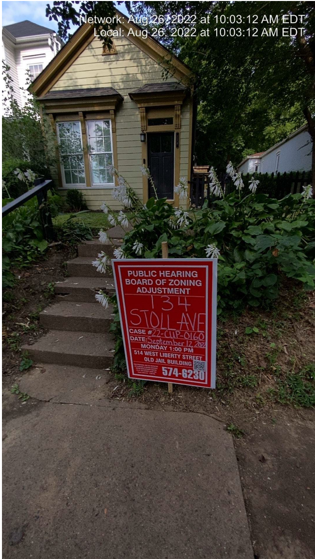
Front of subject property (Google Street view)
