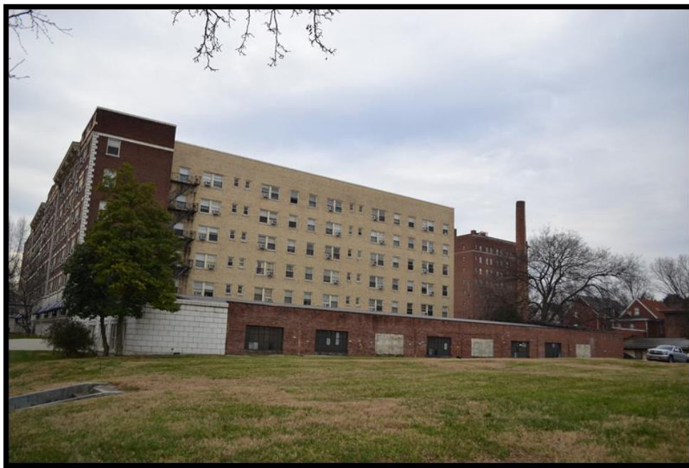
Figure 18. North elevation, looking southwest.
