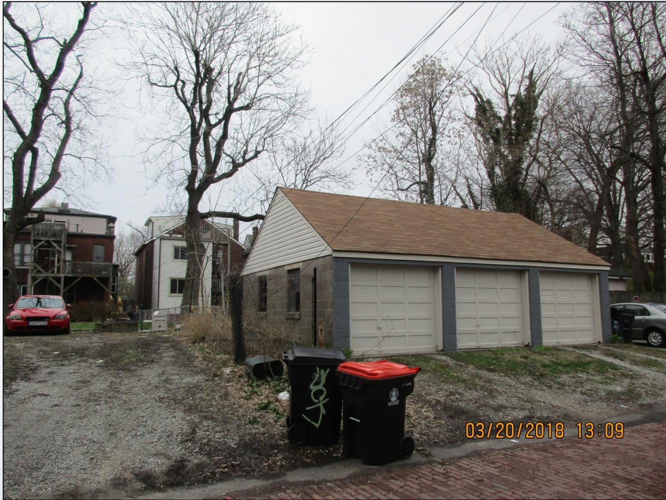
The garage in the rear of the subject property.
